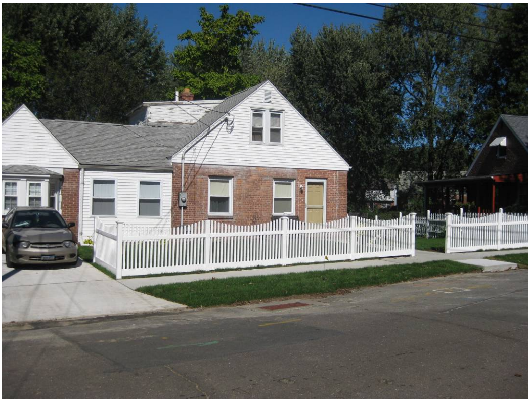
Looking northwest from across Prospect Lane at full restored property.
