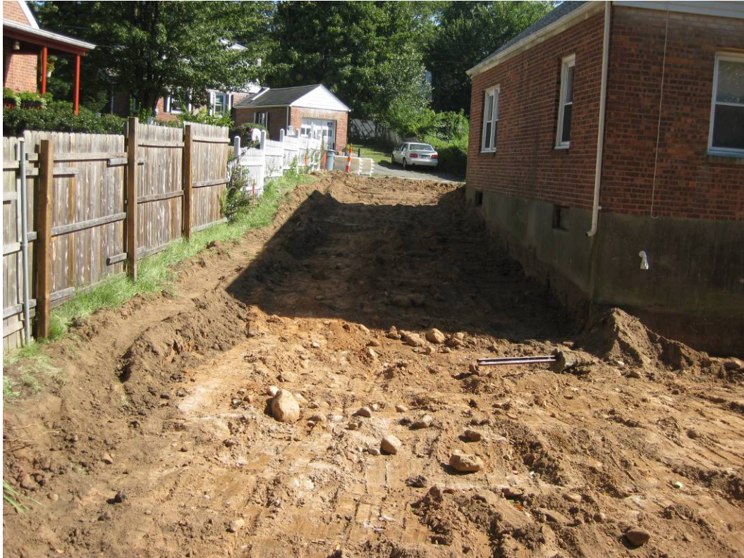
View looking southeast at excavation in side yard.
