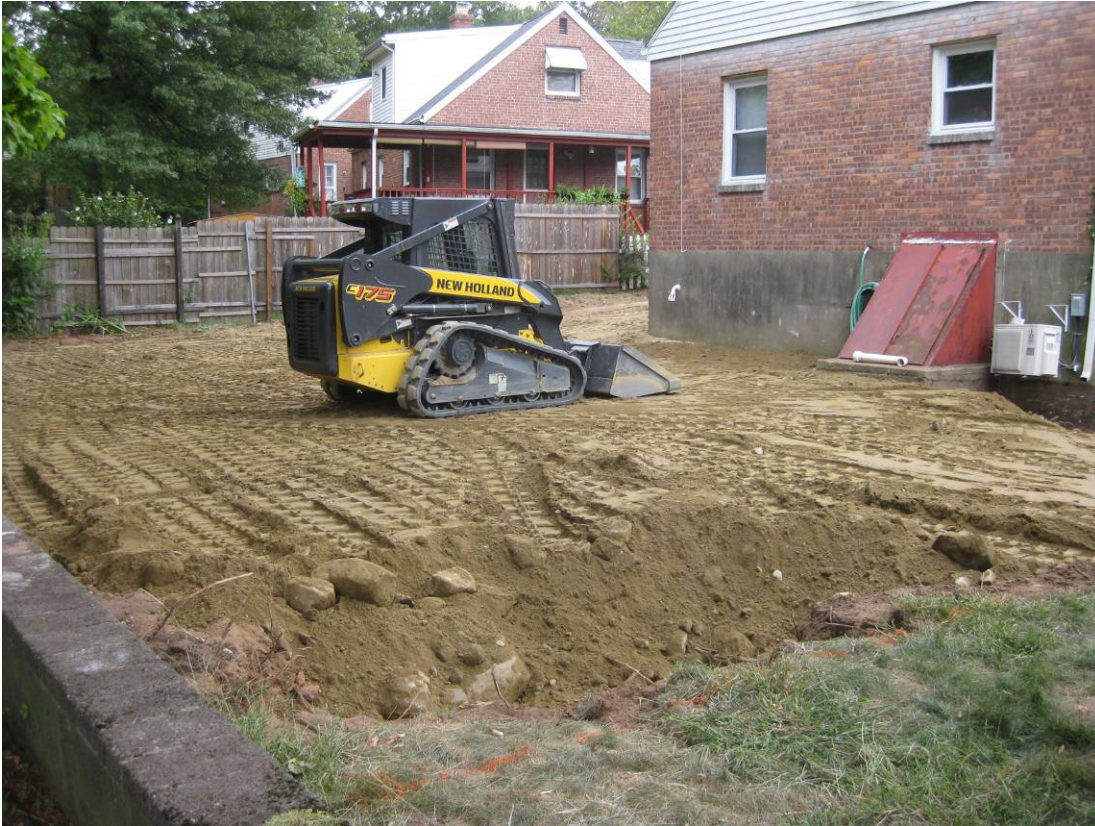
View looking northeast at backfilled back yard.
