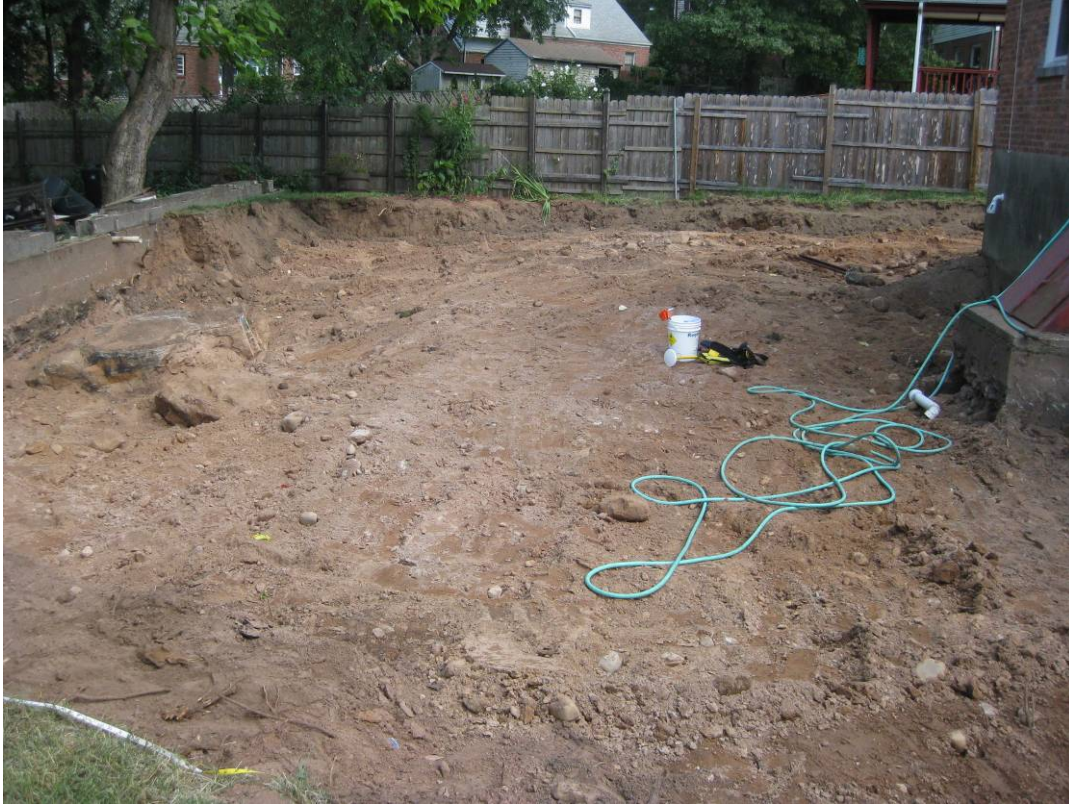
View looking northeast at excavation in back yard.
