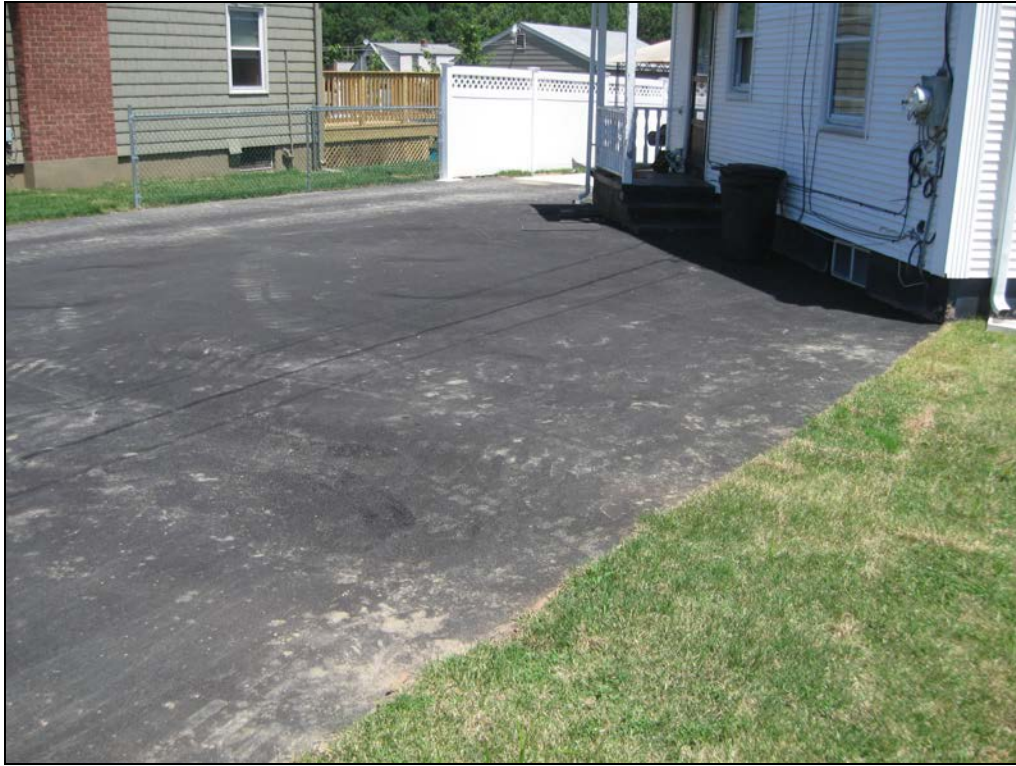
View looking northeast at restored driveway.
