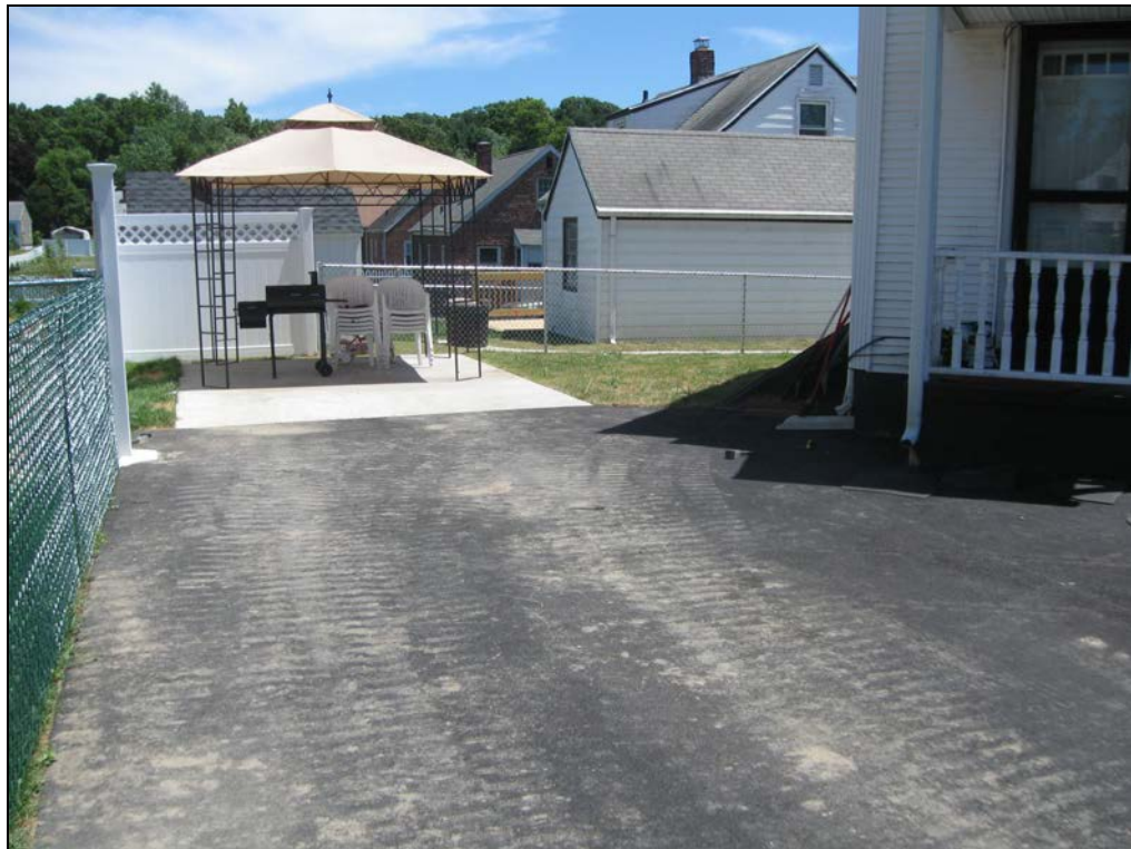
View looking southeast at restored back yard.
