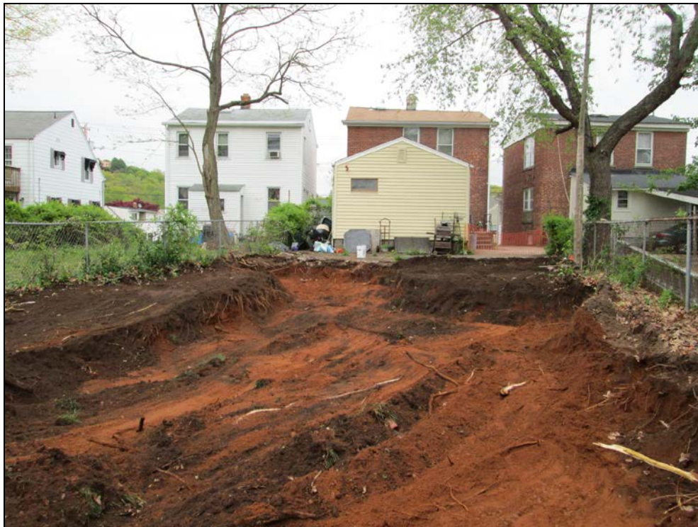
View looking east towards house at excavated back yard.
