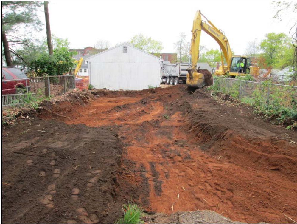
View looking west at excavation in back yard.
