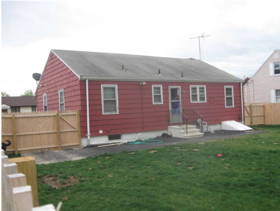
View looking southwest during the Spring 2012 inspection.
