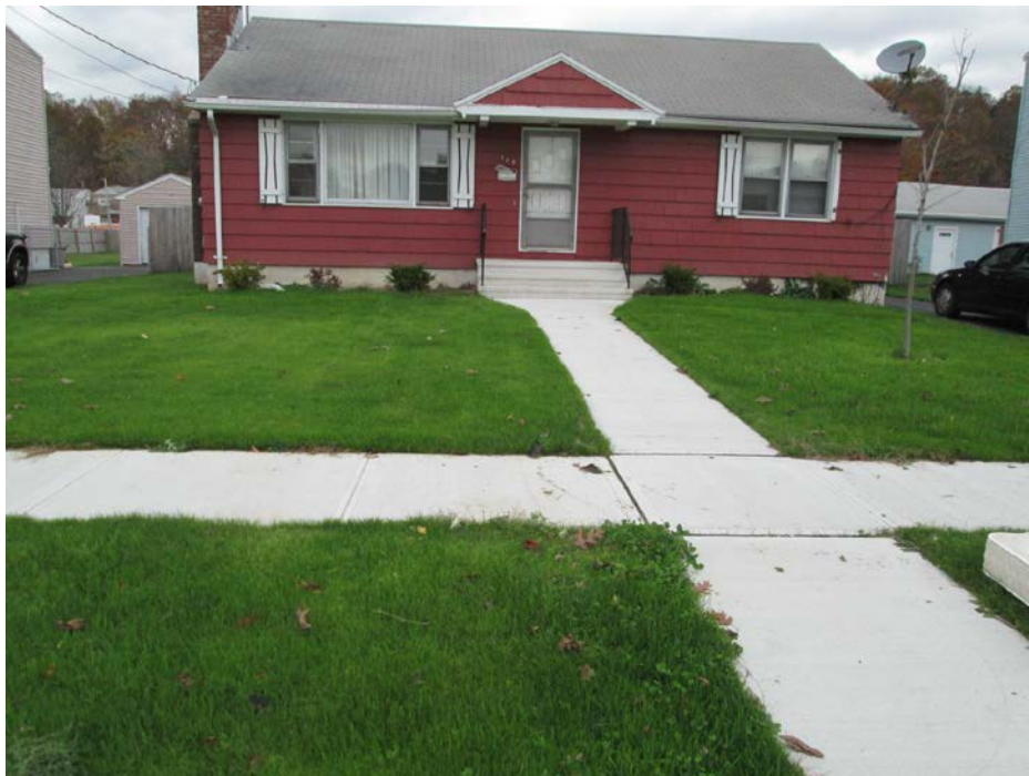
View looking north during the Fall 2012 inspection.
