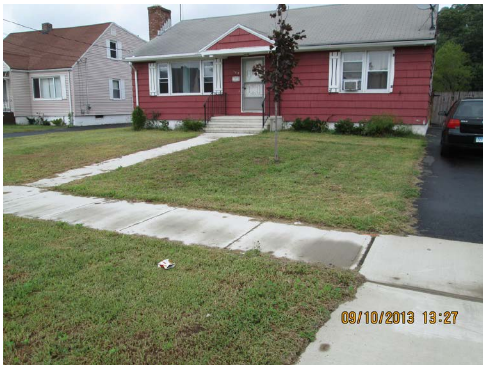
View looking northwest during the Fall 2013 inspection.
