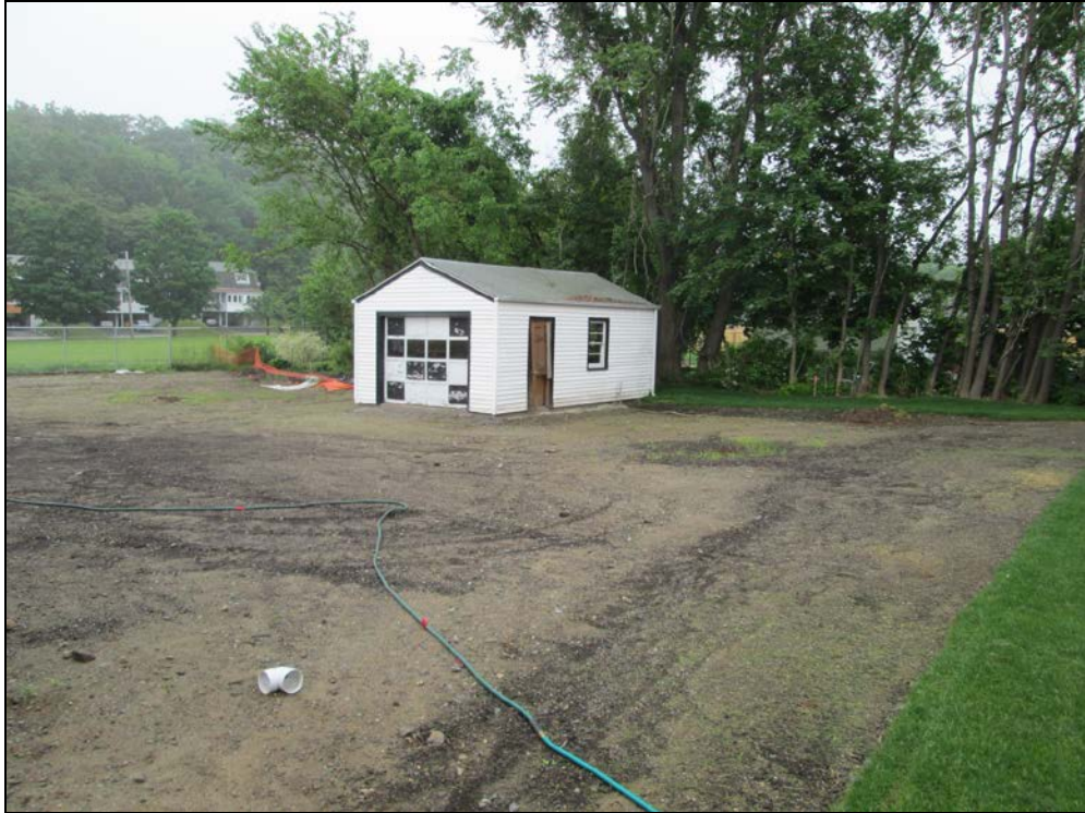
View looking northeast at backfilled back yard.
