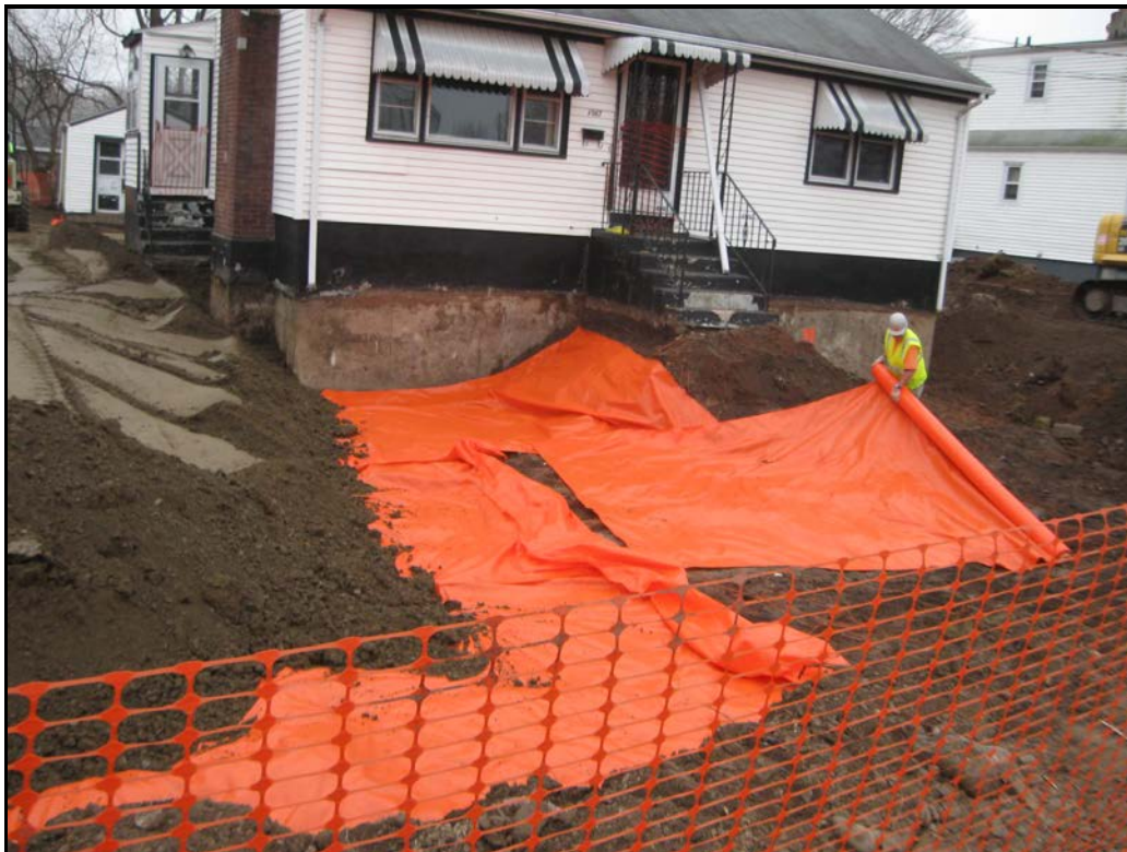
View looking east at partially backfilled front yard with marker barrier over remaining fill.
