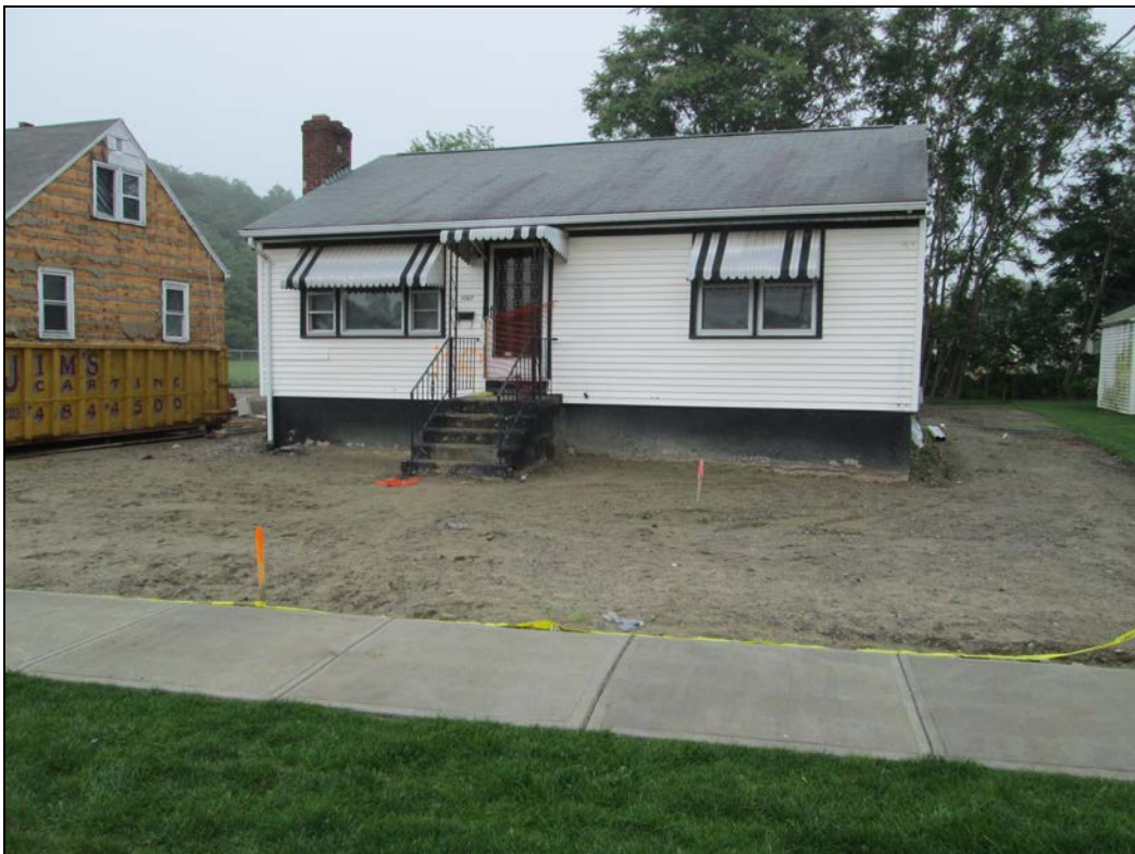
View looking east at backfilled front yard.
