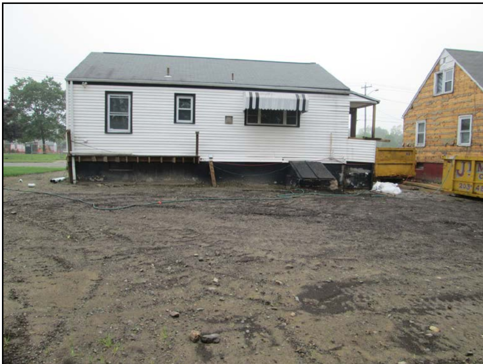
View looking west at backfilled back of 1067 Winchester Avenue.
