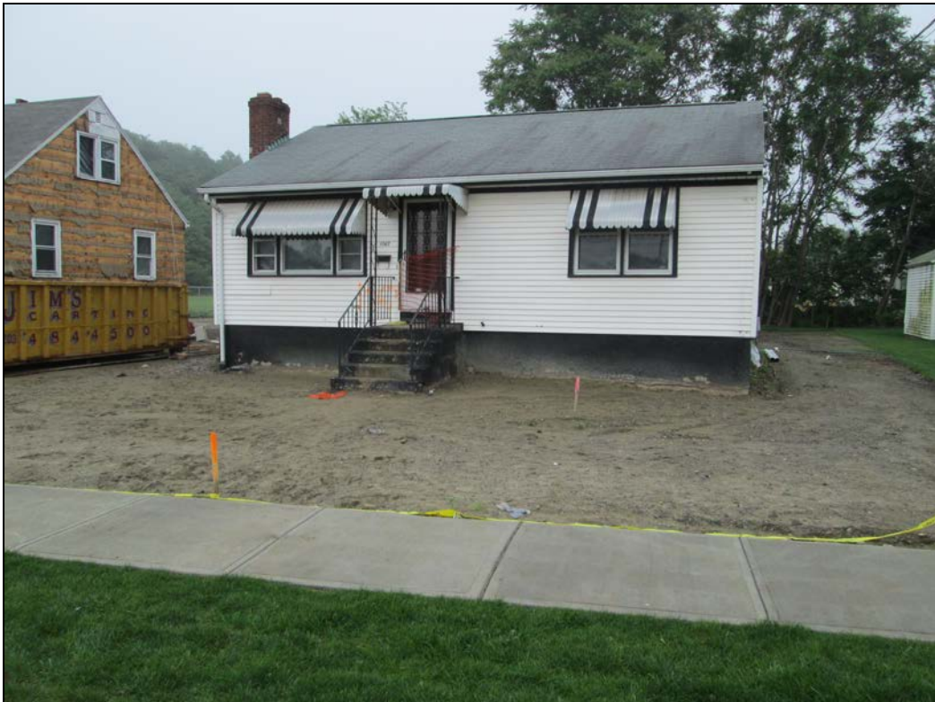
View looking east at backfilled front yard.
