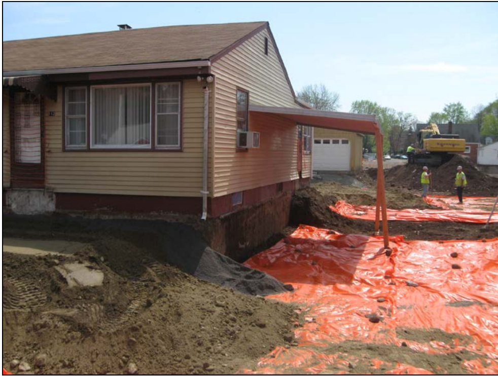
View facing south at excavated side yard under car port.
