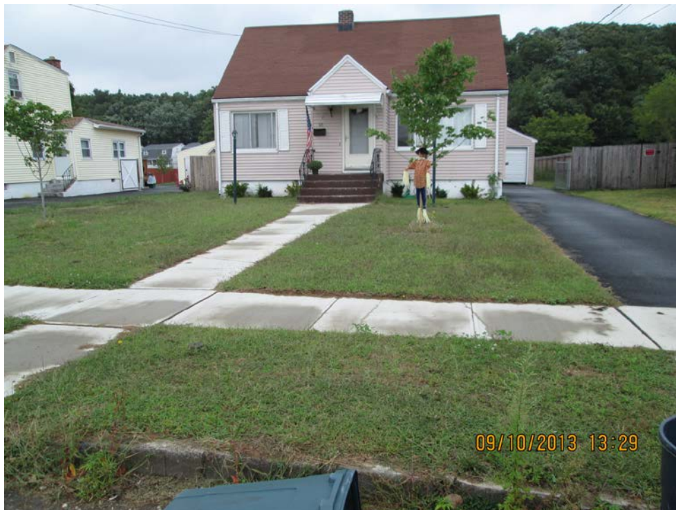
View looking north during the Fall 2013 inspection.
