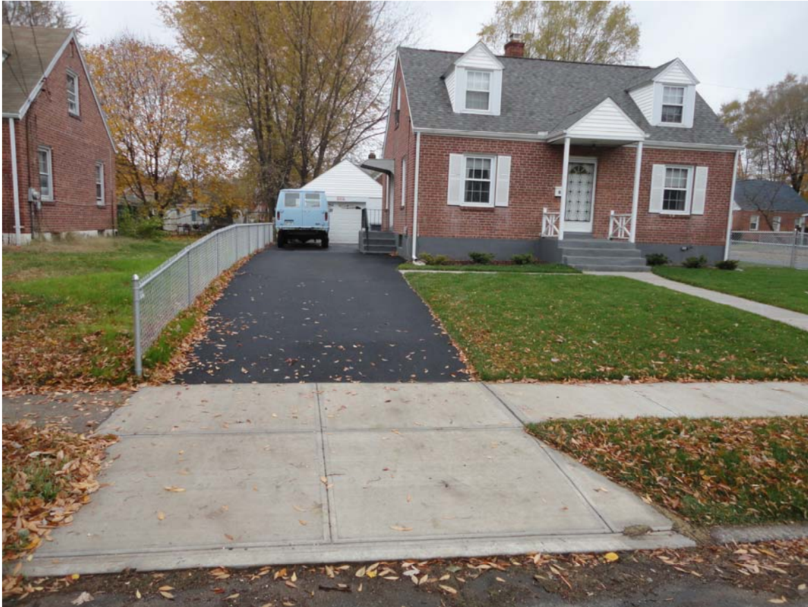
View looking south from Morse Street showing restored driveway, front lawn, and sidewalk.
