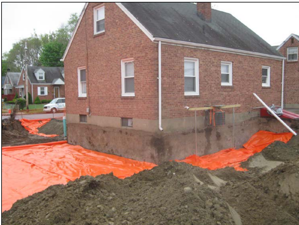
View looking southwest at partially backfilled side and back yard.
