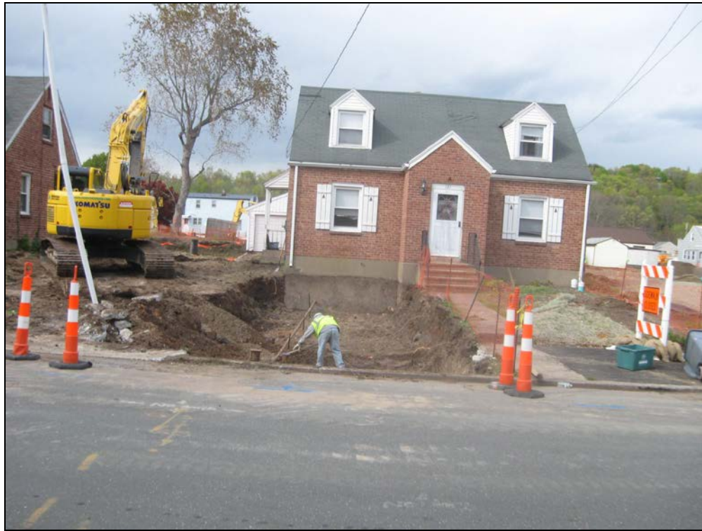
View looking north at partially excavated front yard.
