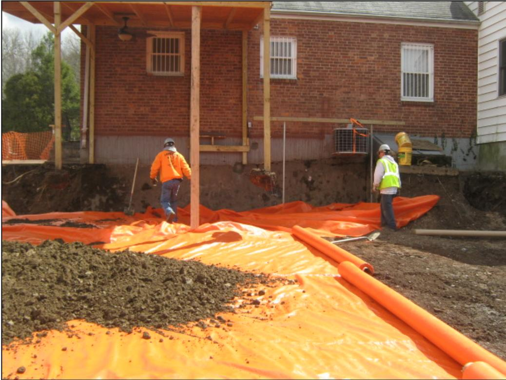
View looking east at marker barrier being installed around back of the house.
