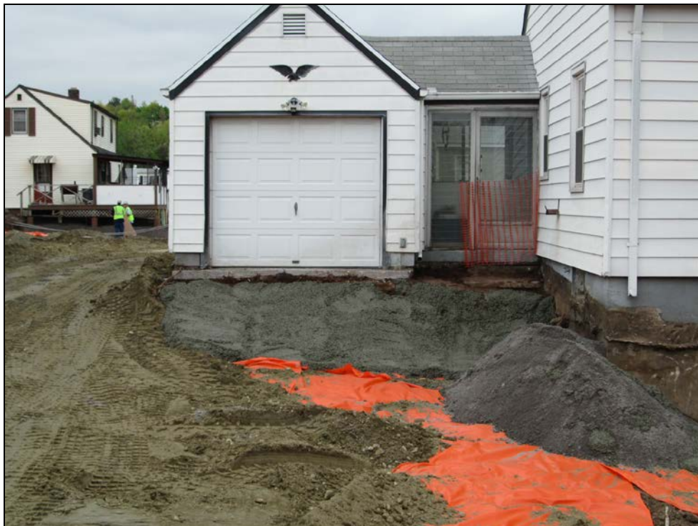
View looking north at partially backfilled front of garage.
