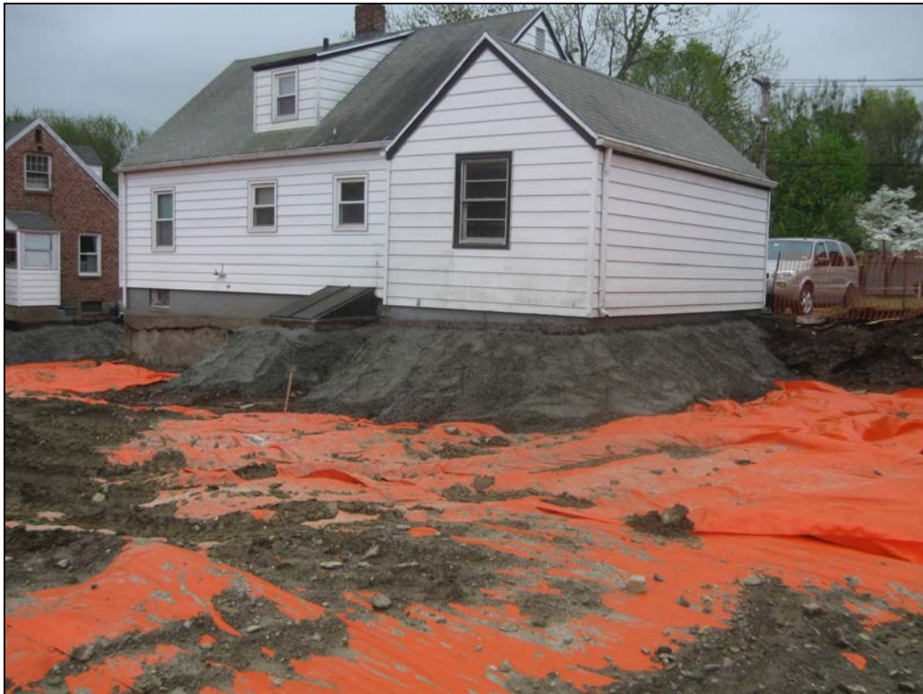
View looking southeast at marker barrier over remaining fill.
