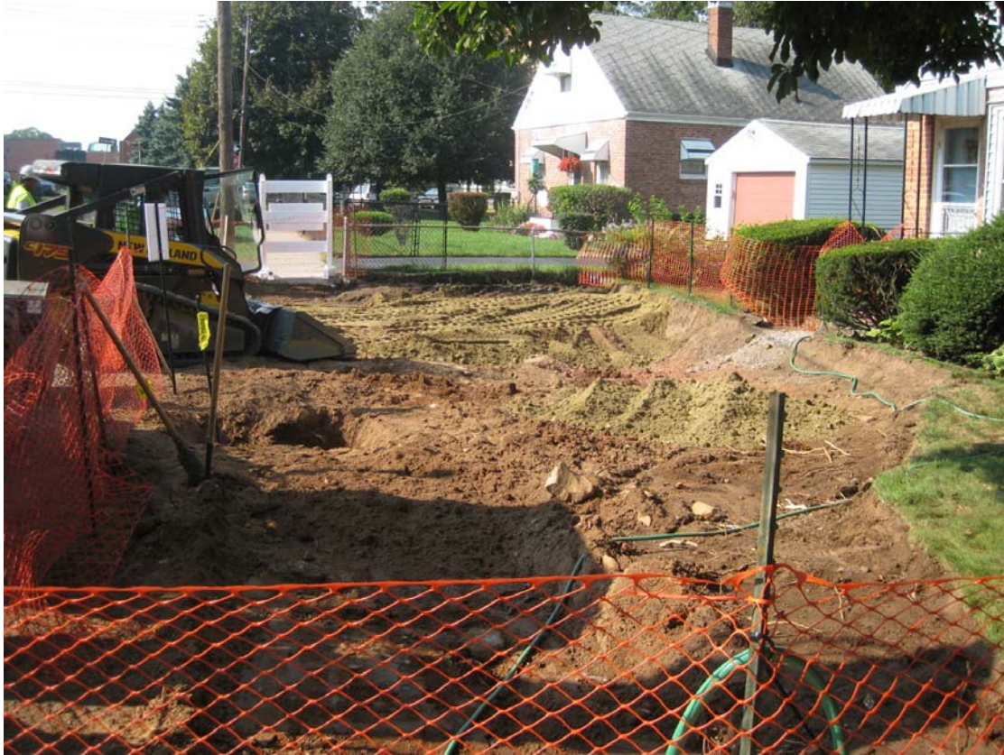
View looking southwest from driveway showing excavation activities in front yard.
