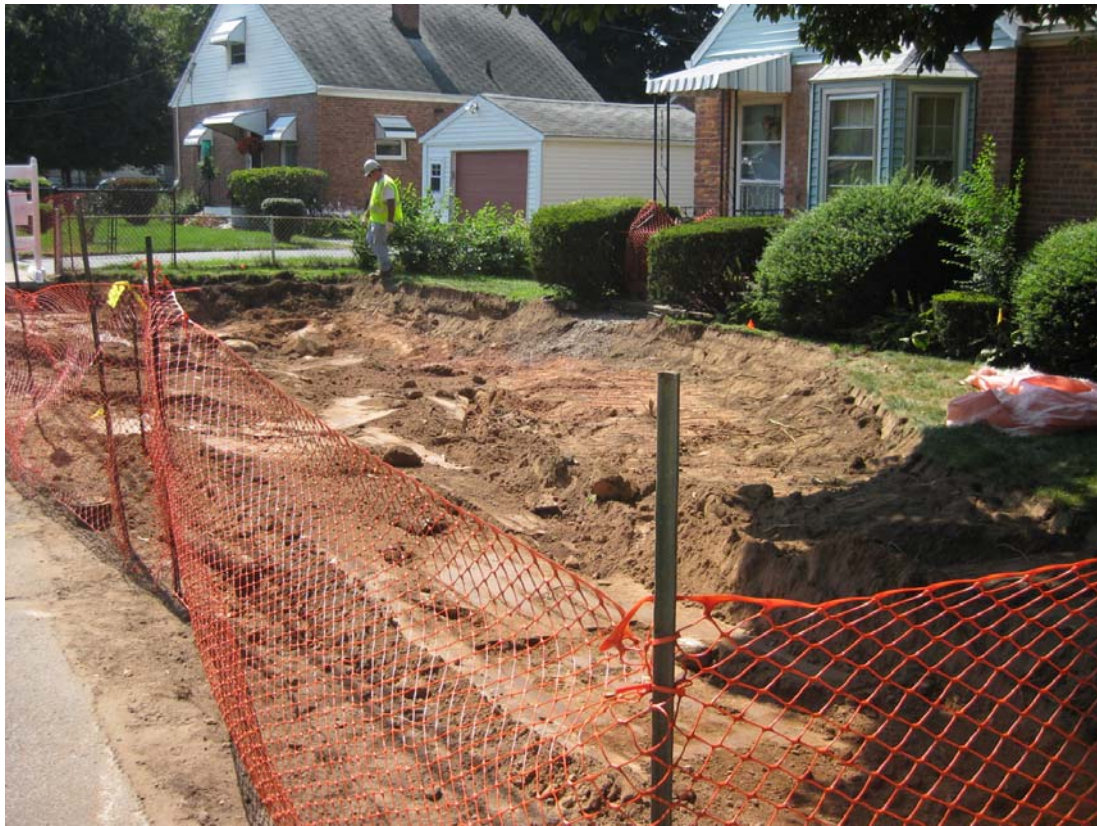
View looking southwest from Prospect Lane showing extent of excavation.
