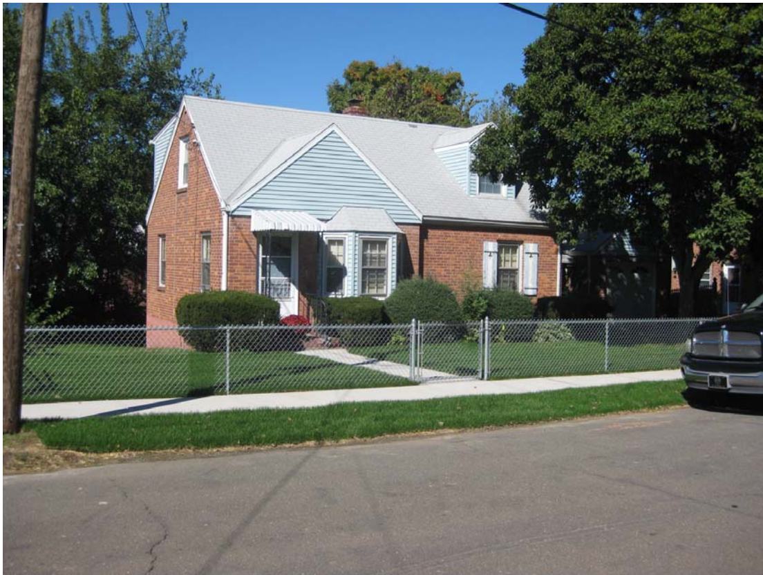
View looking west from across Prospect Lane showing fully-restored property.
