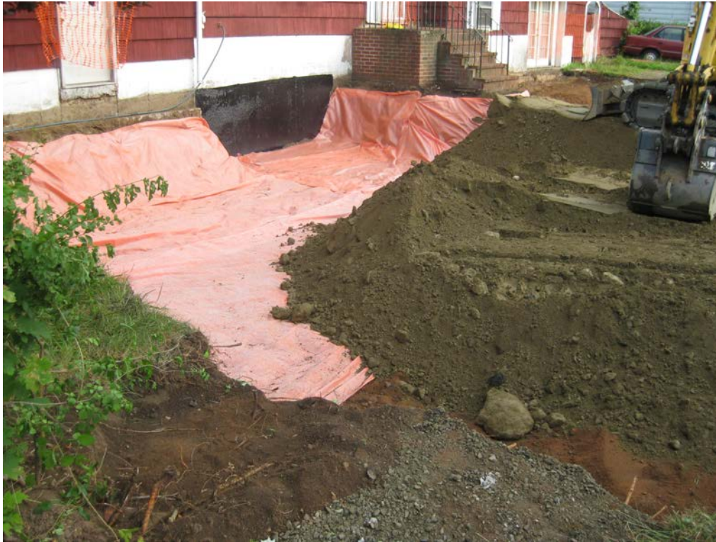
View looking Northwest at partially backfilled front yard
