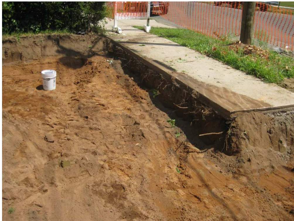
View looking Northeast at excavated front yard
