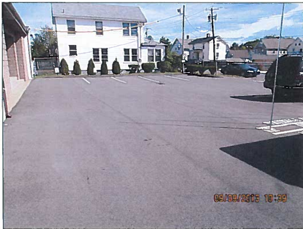
View looking north during Fall, 2013 Inspection.
