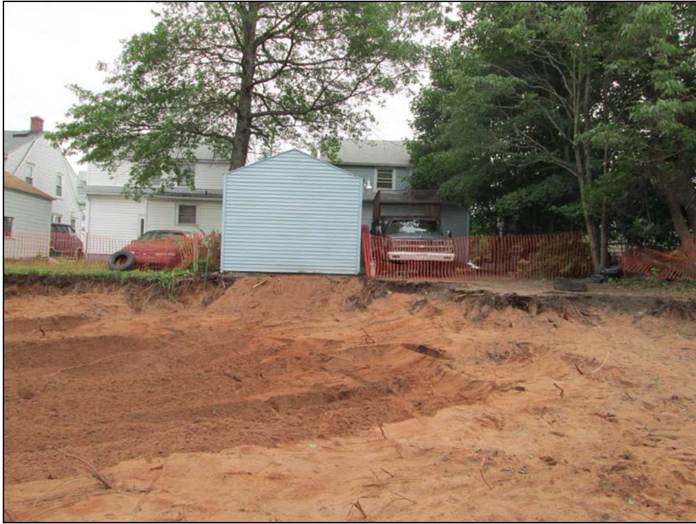
View looking north at extent of excavation in back yard.
