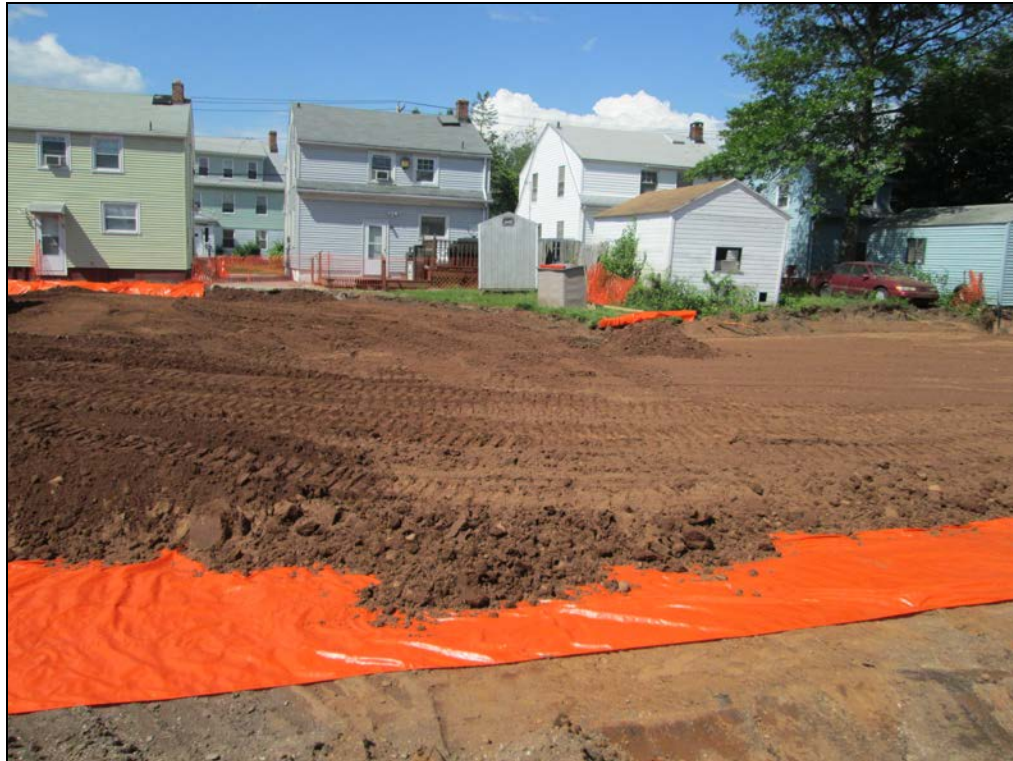
View looking south at partially backfilled back yard.
