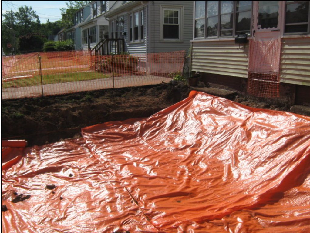
View looking east at front yard following placement of marker barrier.
