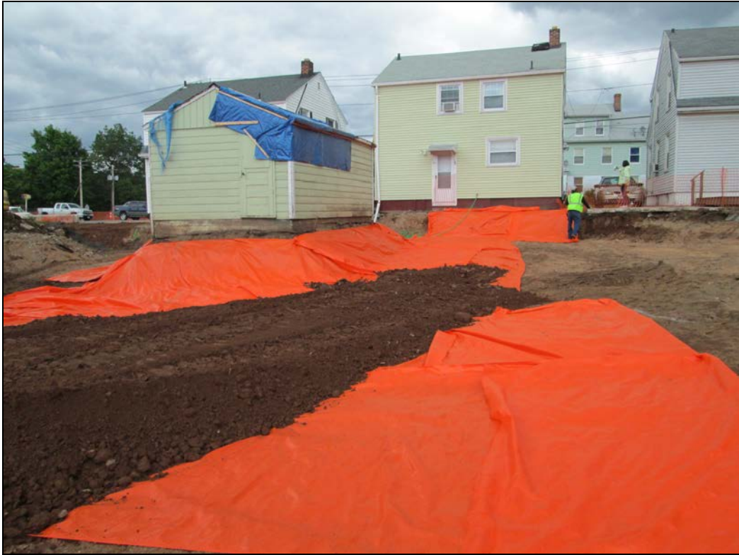
View looking north at excavated back yard.
