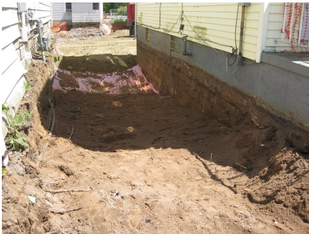
View looking East at excavated side yard
