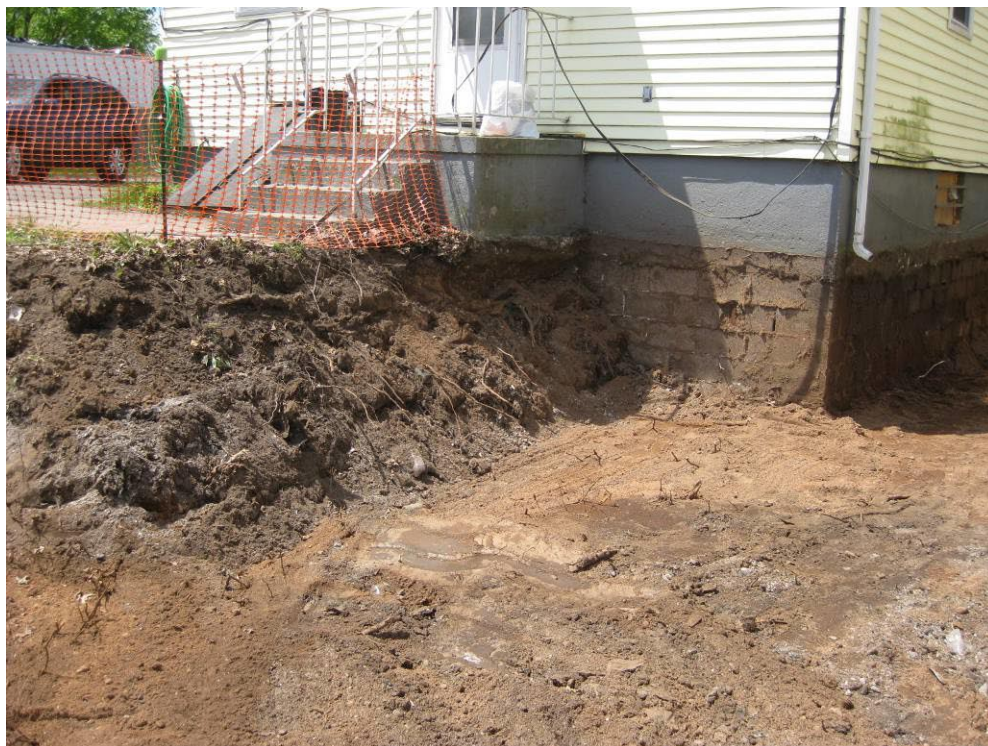
View looking Southeast at excavation around back entrance
