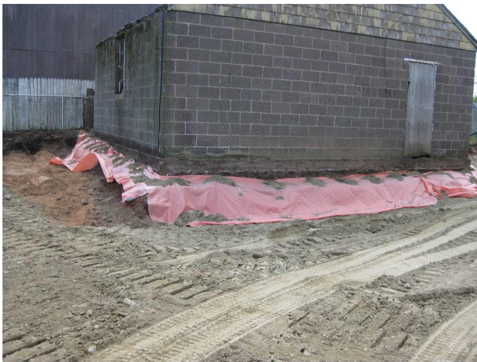
View looking South at excavation around garage
