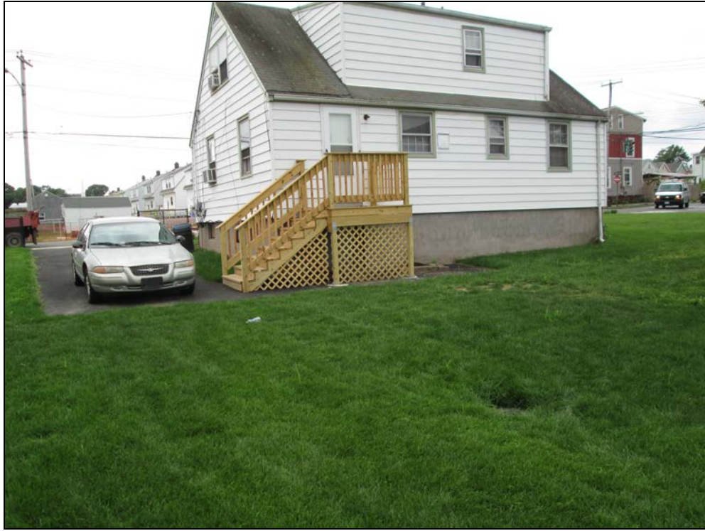
View looking south at restored back yard.
