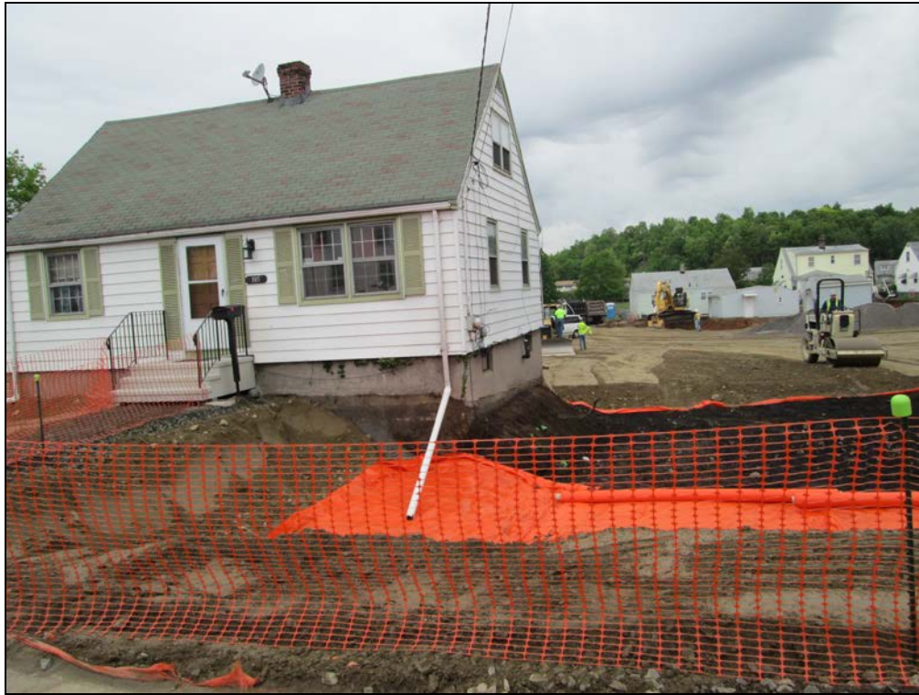
View looking north at partially backfilled front yard.
