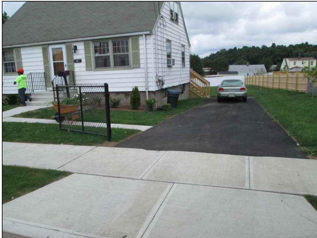
View looking north at restored front yard.
