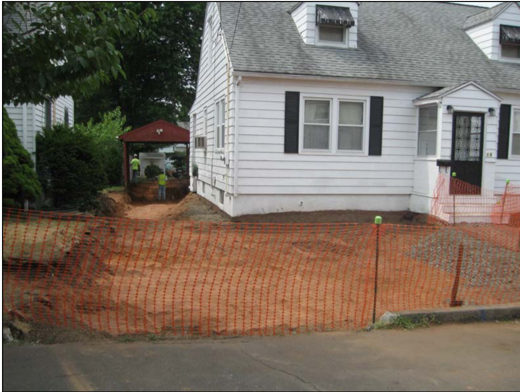
View looking south at excavated driveway area.
