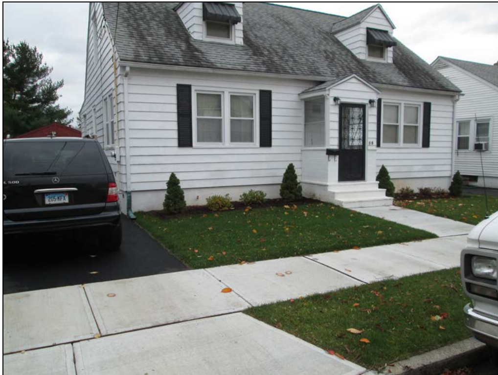
View looking south at restored front yard.
