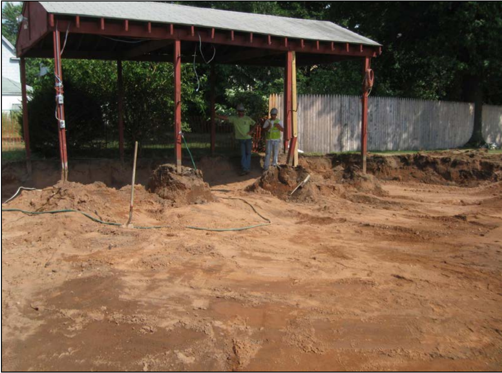
View looking southeast at excavated carport area.
