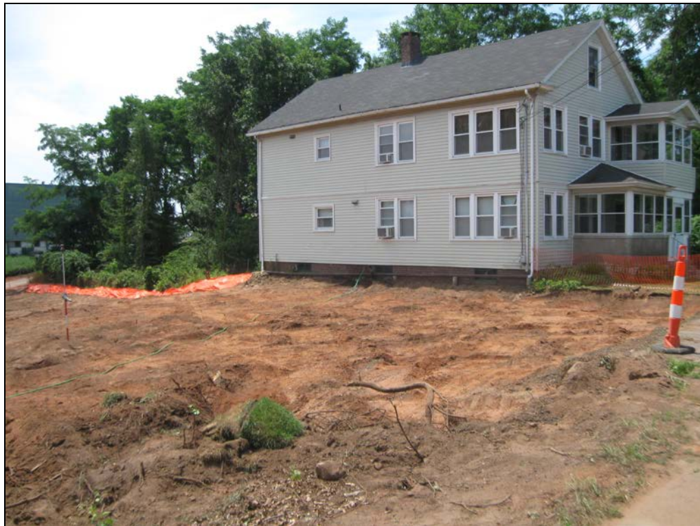
View looking southwest at excavated side yard.
