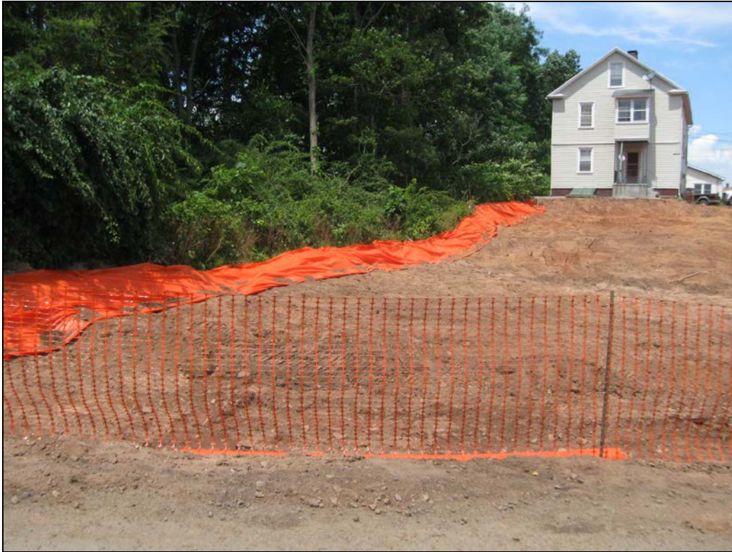
View looking north at excavated back yard.
