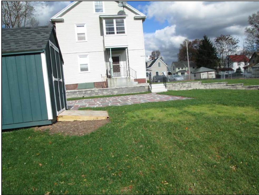
View facing north at restored back yard.
