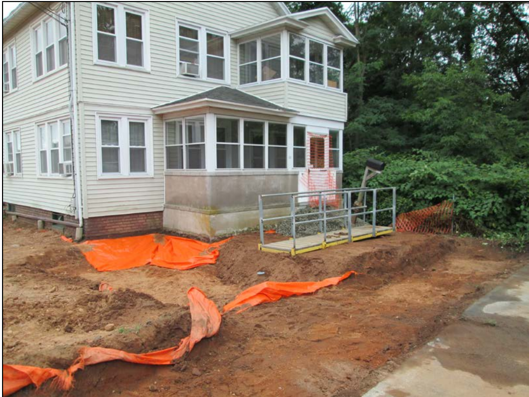
View looking southwest at partially backfilled front yard.
