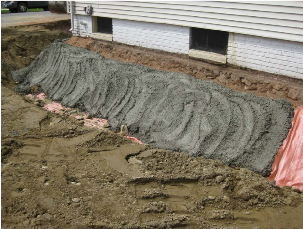
View looking Northwest at side yard
