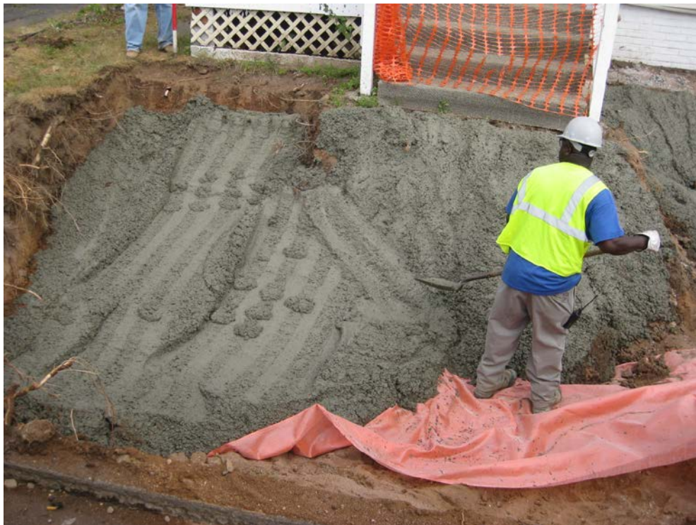
View looking East at front steps with concrete
