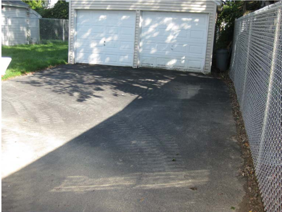
View looking East at restored driveway
