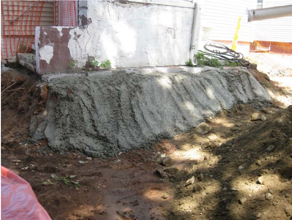
View looking West at concrete along back steps
