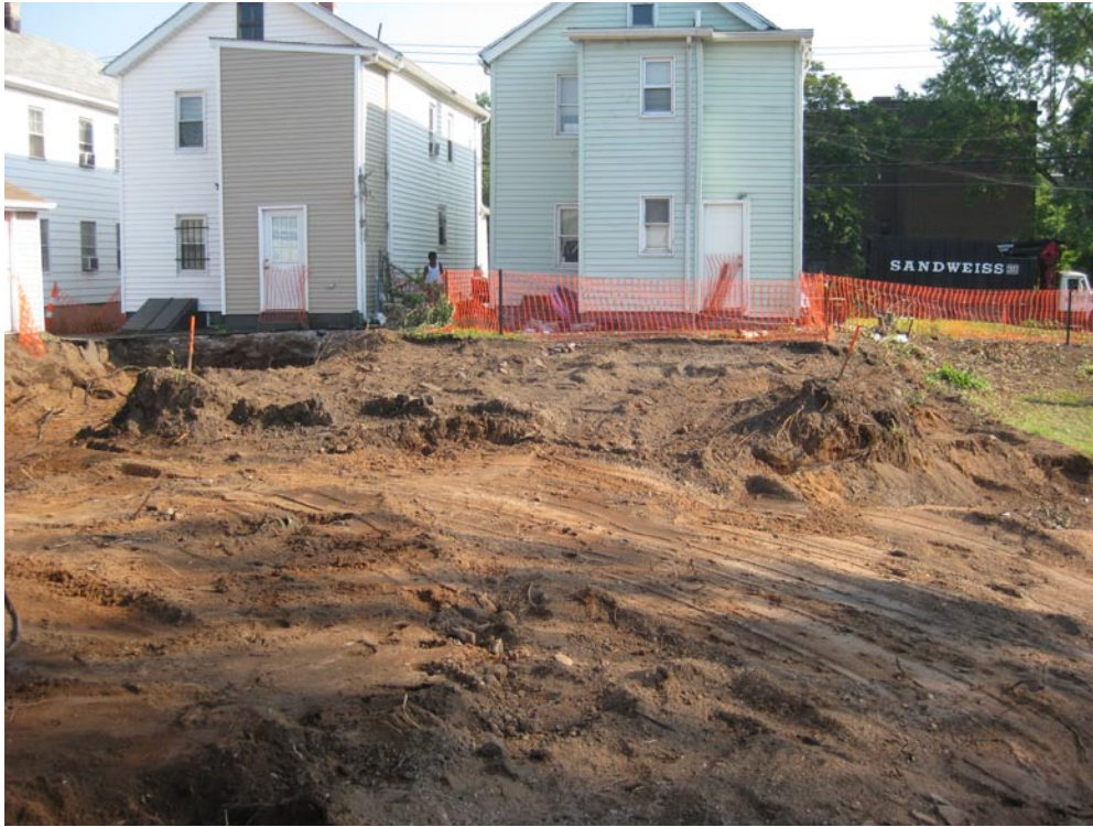
View looking North at excavated backyard
