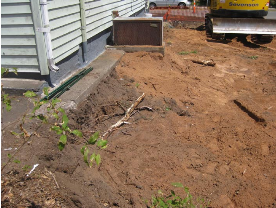
View looking North at excavation area along side of house
