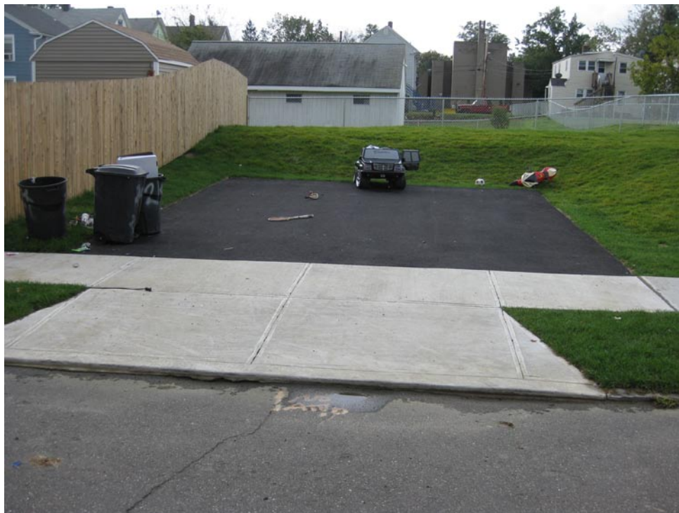
View looking South at restored driveway and side yard
