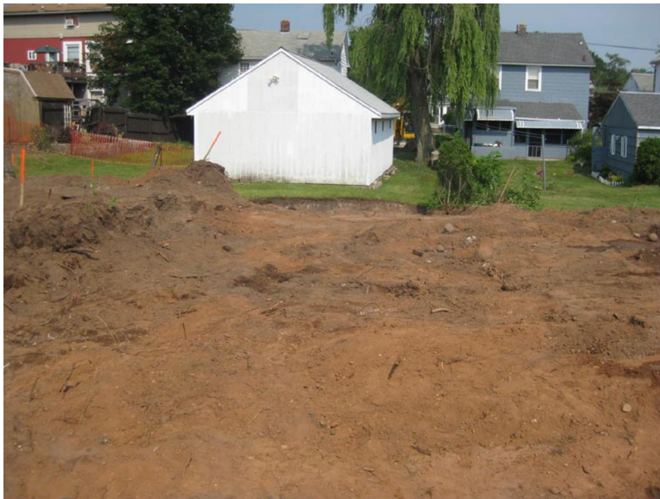
View looking East at excavation of side yard
