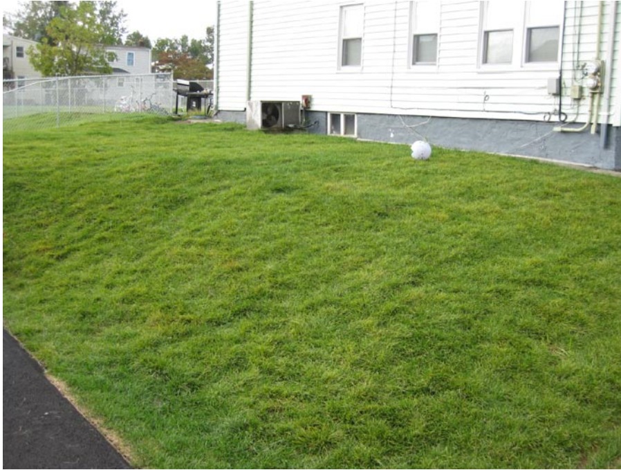
View looking Southwest at restored yard at side of house
