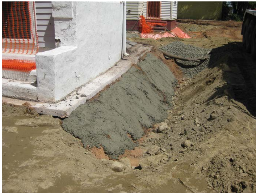
View looking North at concrete along back of house
