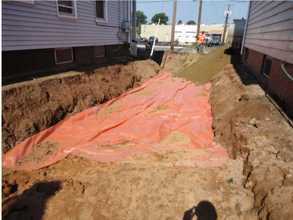
View looking West at excavated side yard with marker barrier
