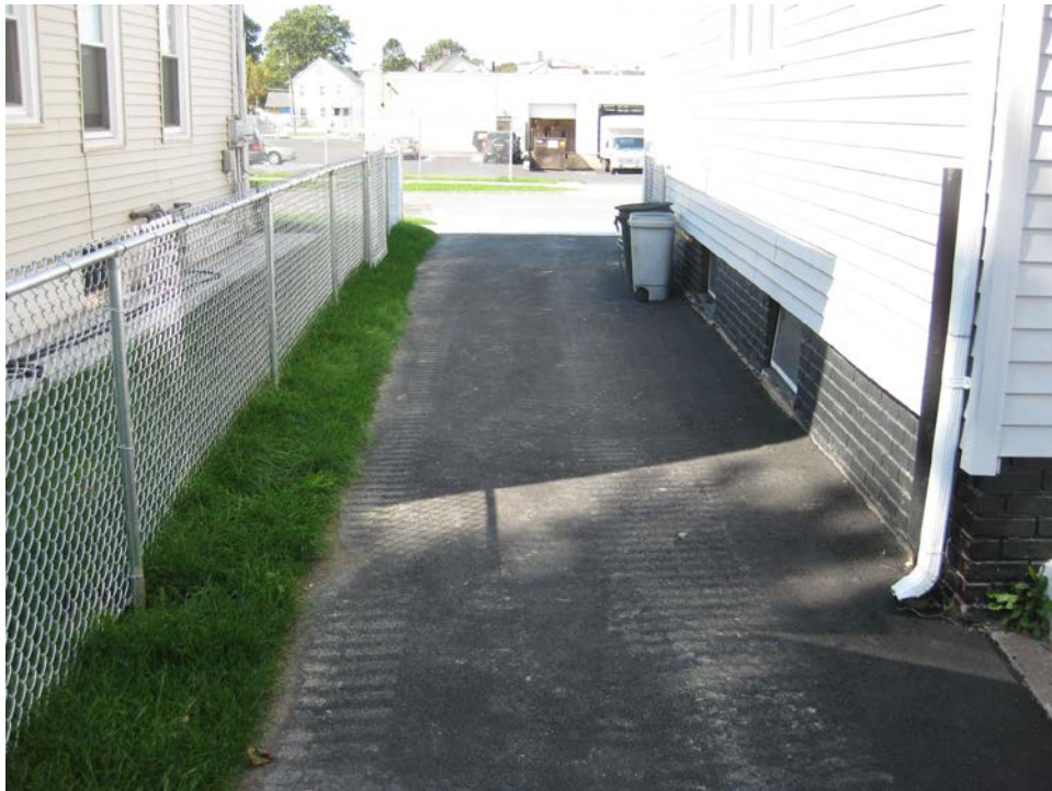
View looking West at restored driveway
