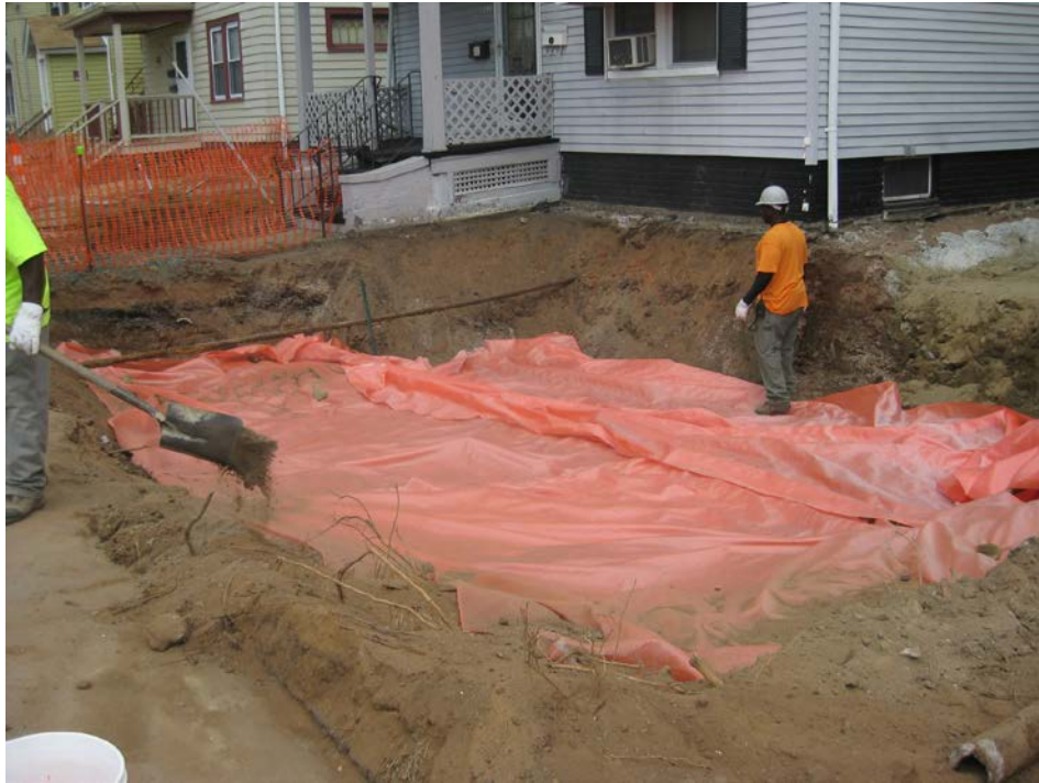
View looking Northeast at marker barriers along side and front of house
