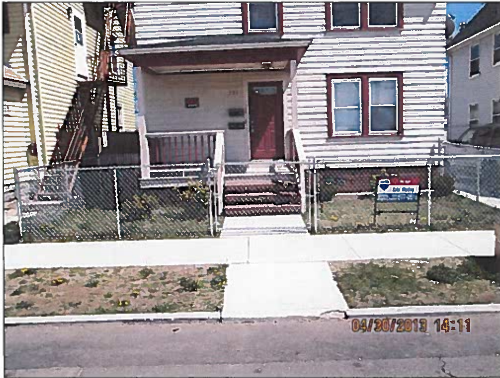
View looking east during the Spring 2013 inspection.
