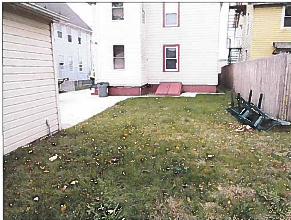
View looking west during the Fall 2012 inspection.
