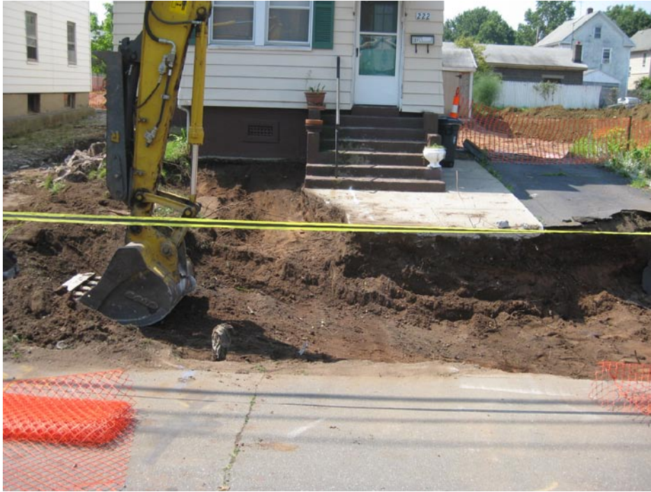
View looking South at excavation in front of house
