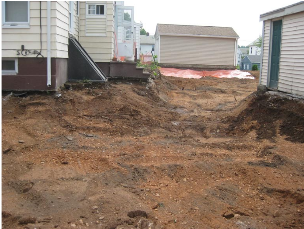
View looking East at excavation area behind house
