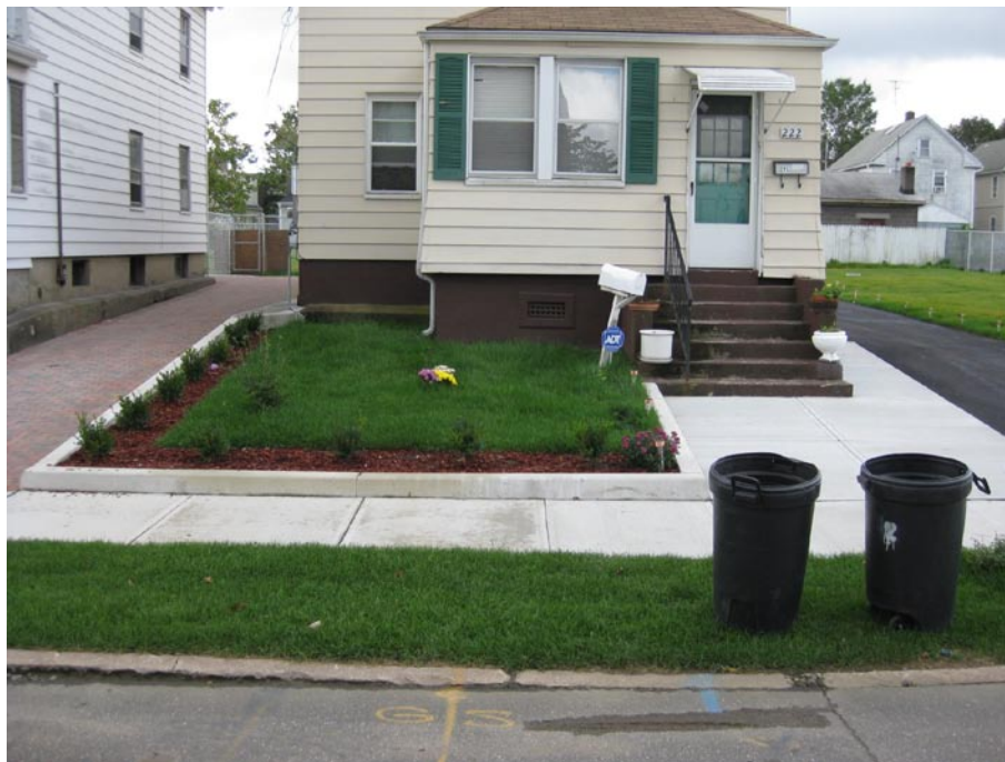
View looking South at restored front of property
