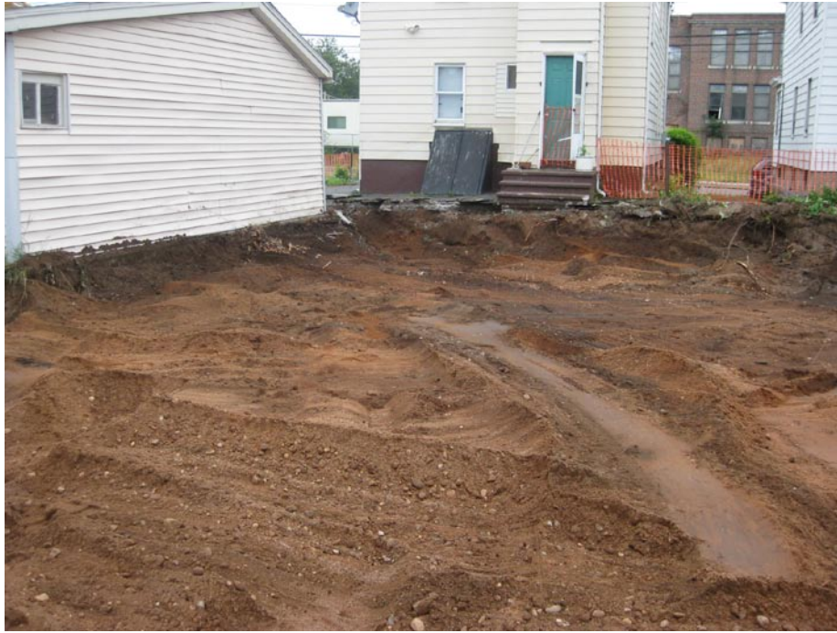
View looking North at excavated back yard
