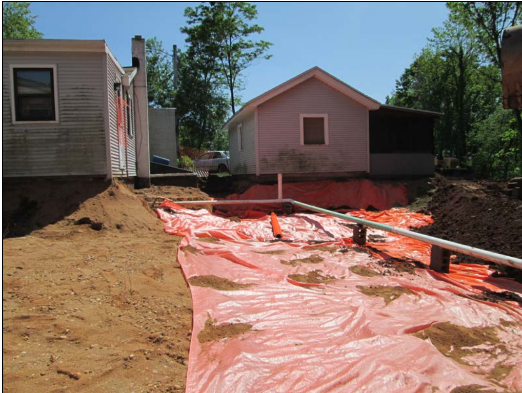
View looking south at excavated yard from the adjacent property.
