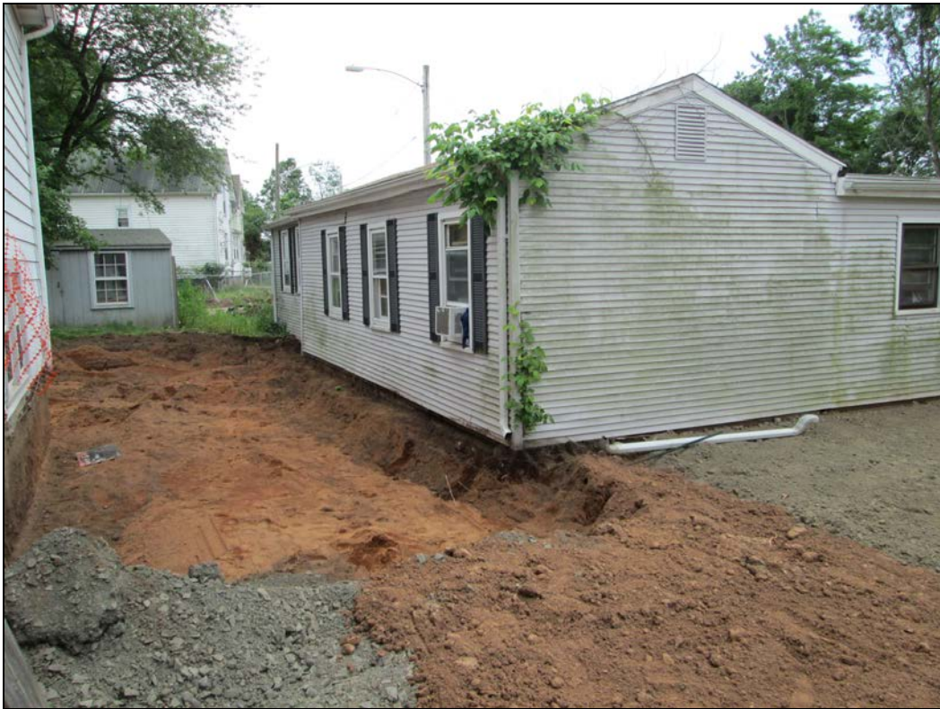
View looking north at excavated back yard.
