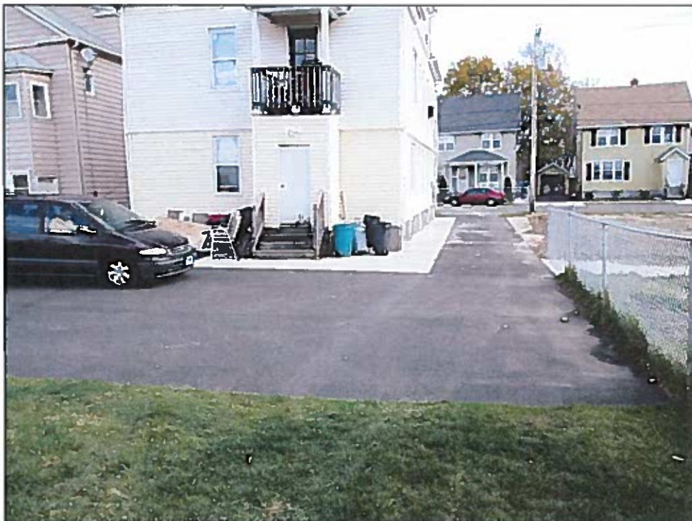
View looking east during the Fall 2012 inspection.
