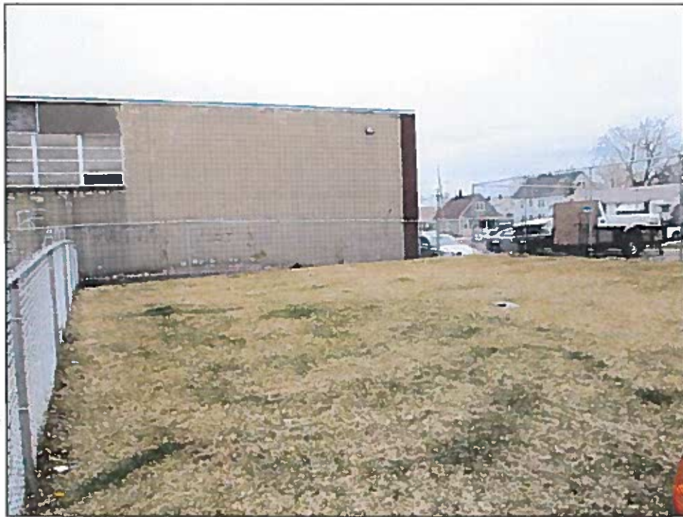
View looking west during the Spring 2013 inspection.
