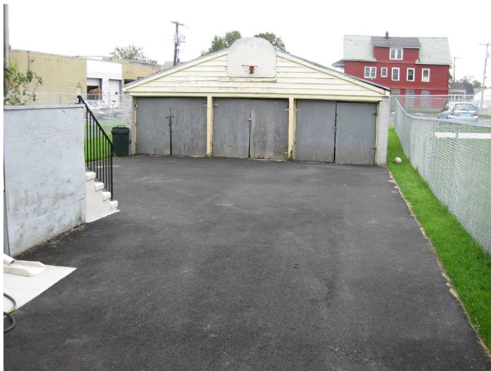
View looking North at restored driveway
