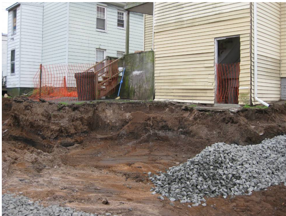
View looking Southeast at excavated back yard
