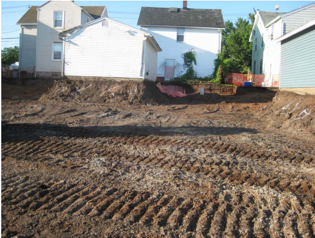
View looking South at excavated back yard
