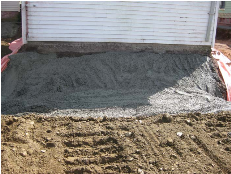
View looking South at concrete marker barrier along back of garage
