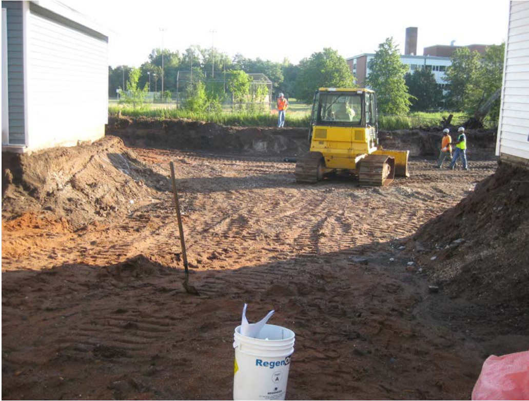
View looking North at excavated back yard
