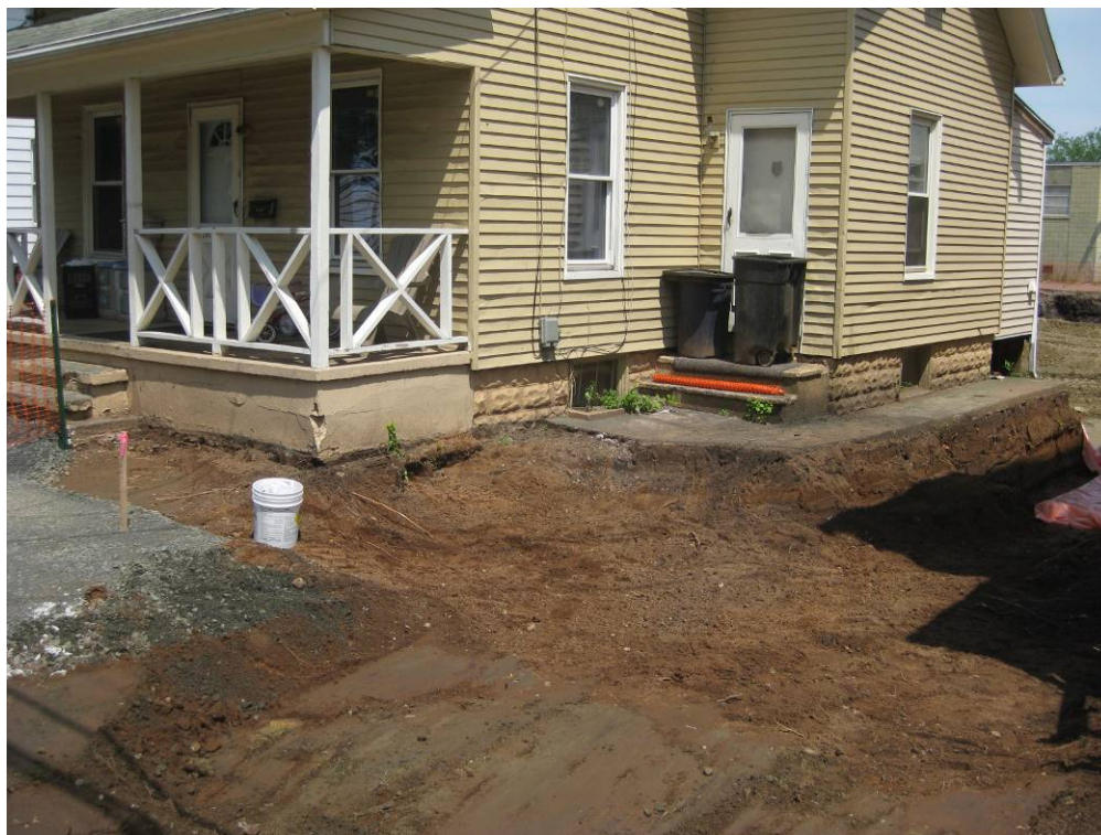
View looking Northwest at excavated side yard
