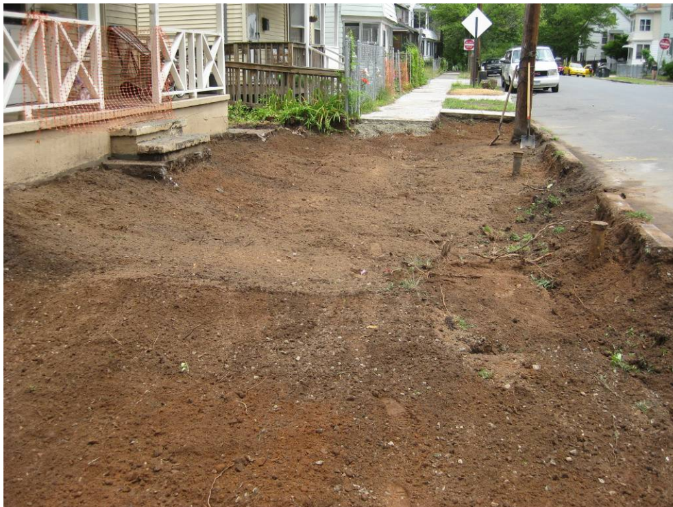
View looking East at excavated front yard
