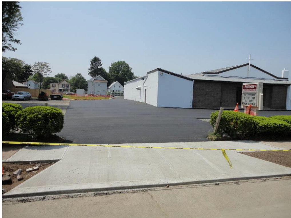
View looking West at restored parking area
