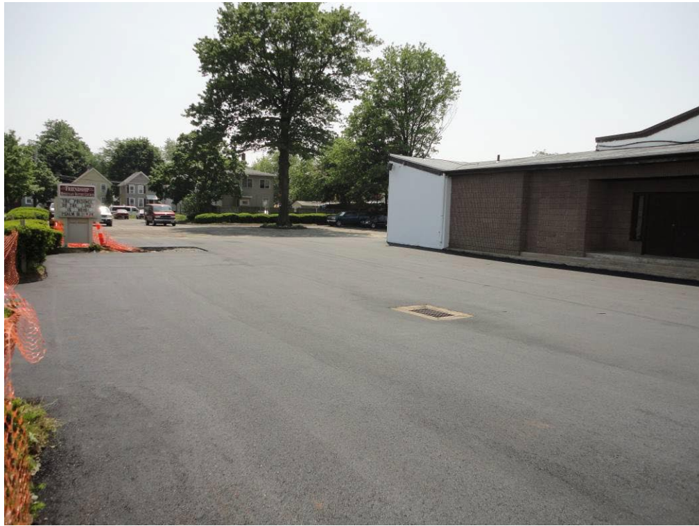
View looking South at restored parking area
