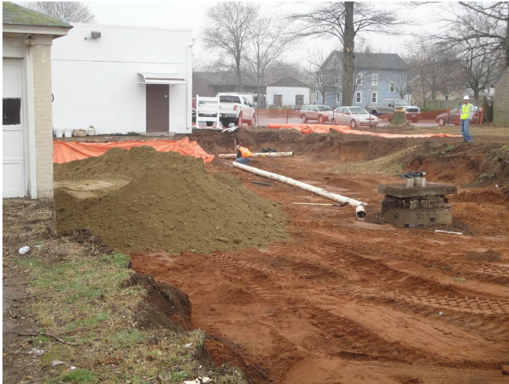
View looking Southeast at excavated catchbasin
