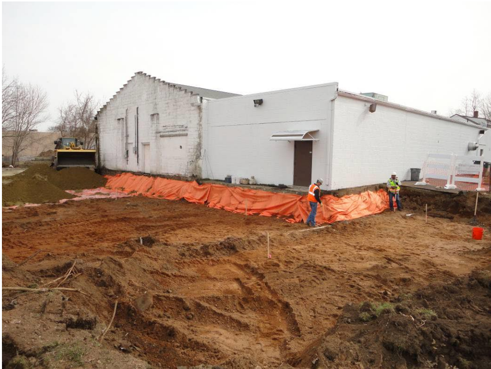
View looking Northeast at partially backfilled property as marker barrier is placed
