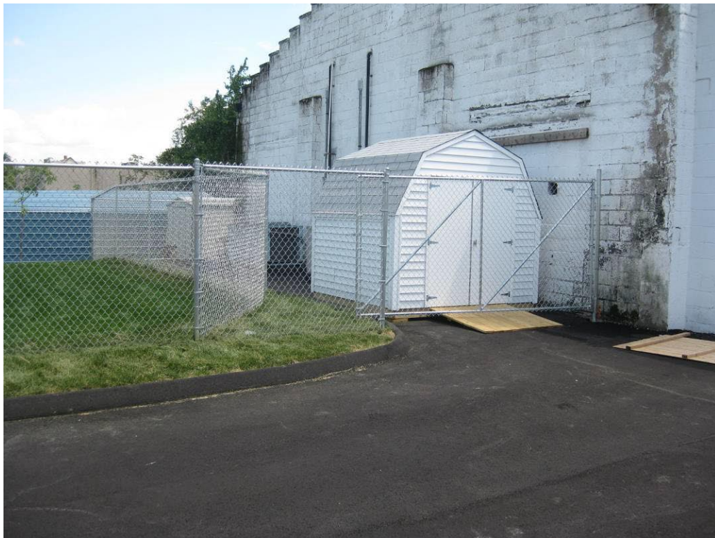
View looking Northeast at restored features
