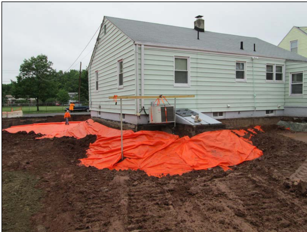
View looking northeast at excavated back yard.
