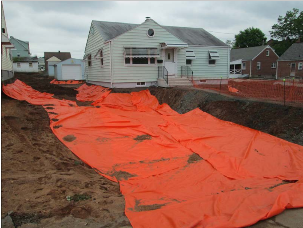
View looking south at excavated front yard.
