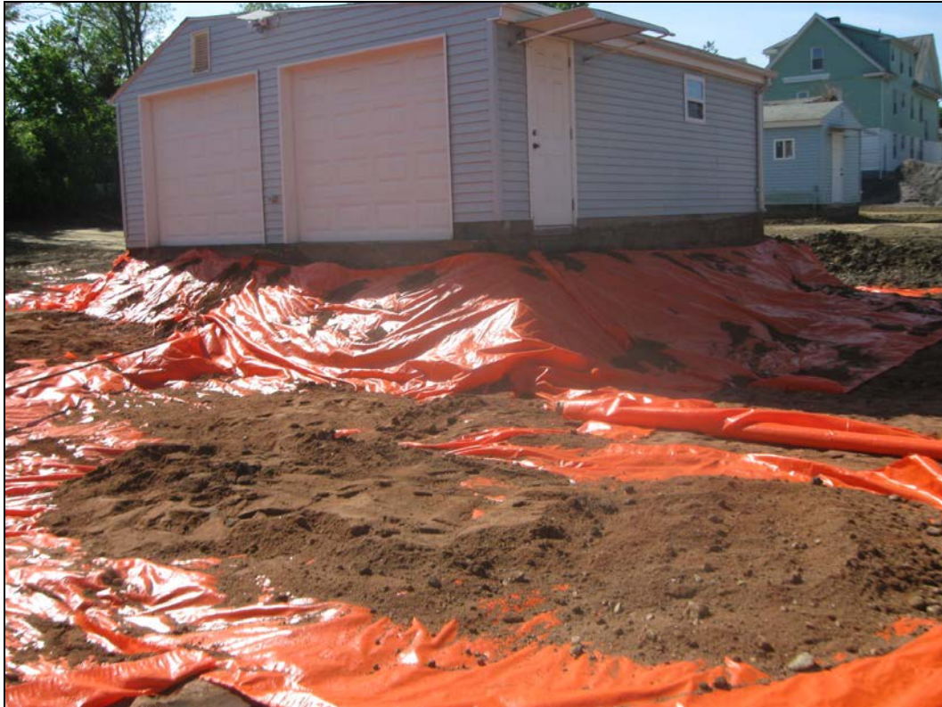
View looking southeast at excavated area around the garage.
