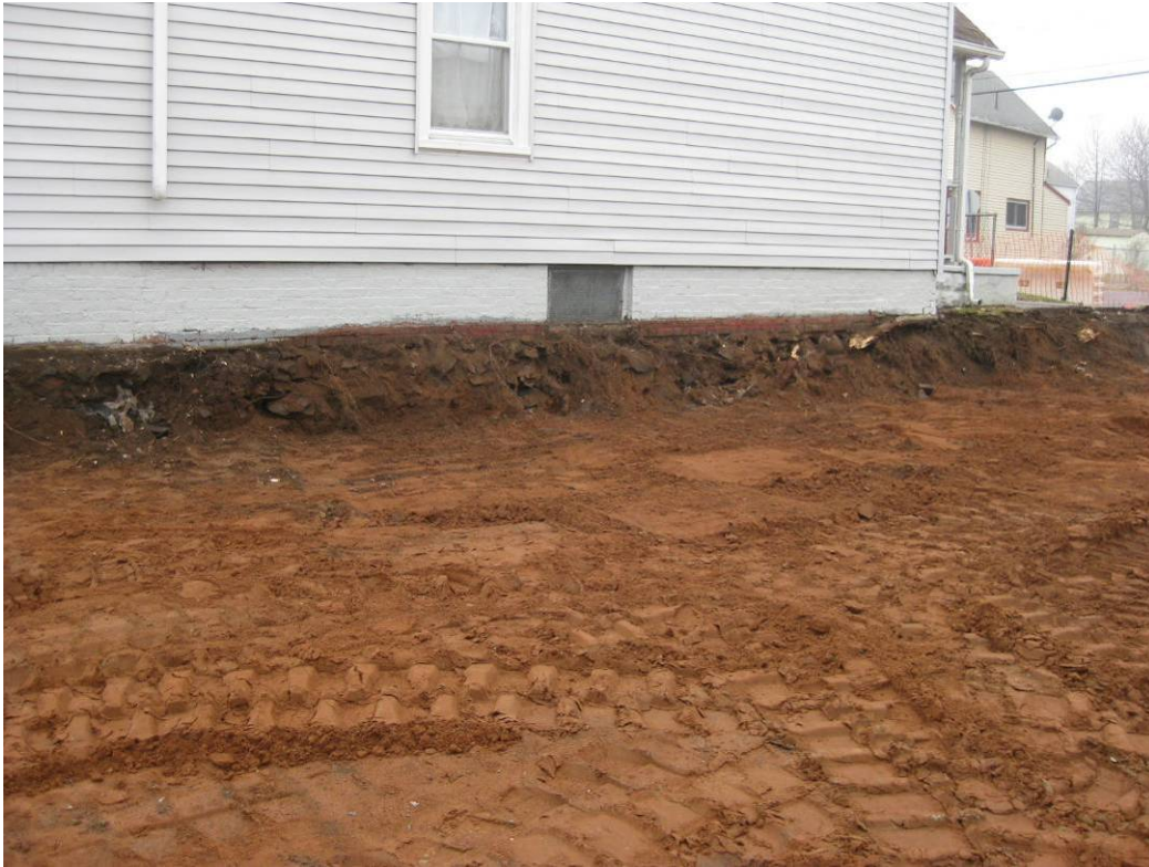
View looking northeast of extent of excavation at former driveway
