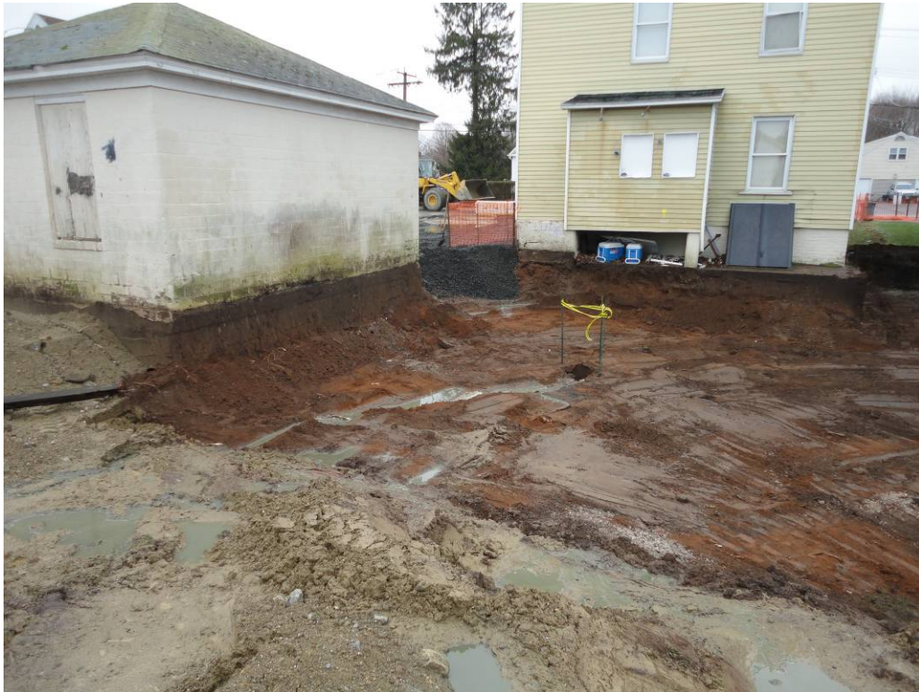
View looking west at extent of excavation in backyard
