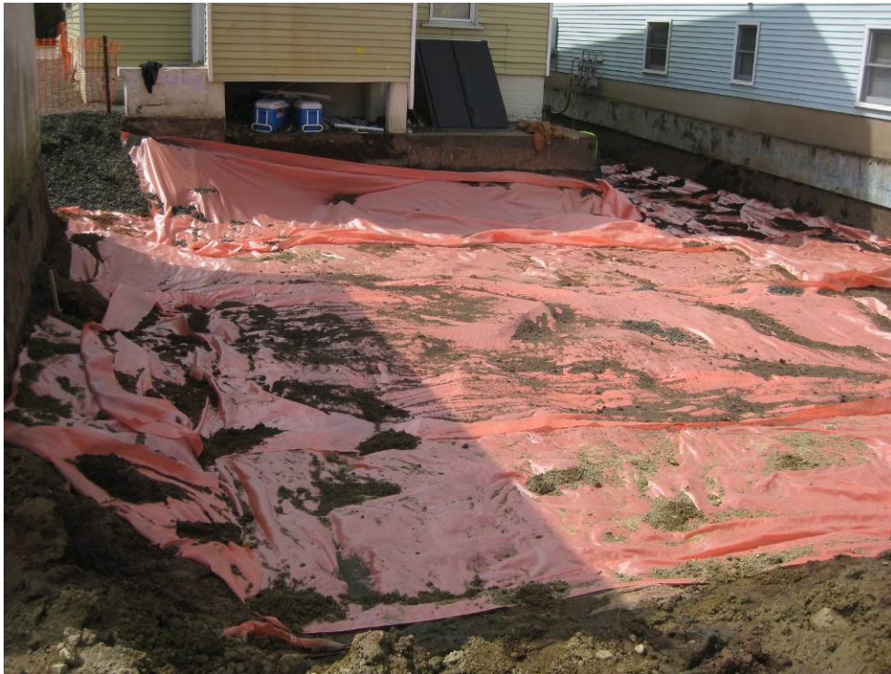
View looking west at filter fabric at base of backyard excavation
