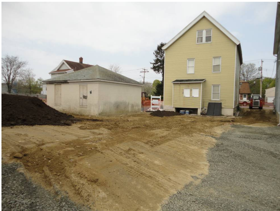
View looking southwest at backfilled excavation
