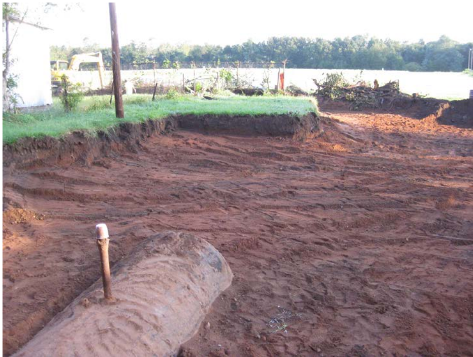
View looking North at excavated back yard
