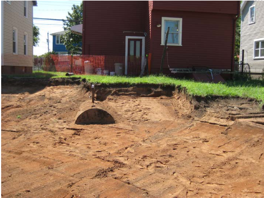
View looking South at excavated back yard and partially exposed UST
