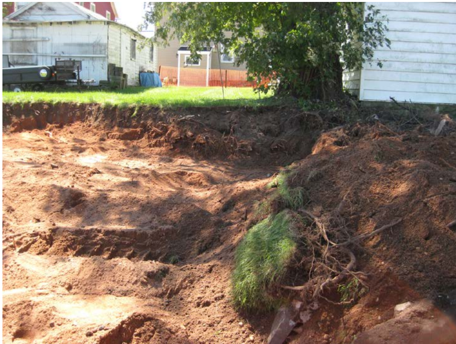
View looking South at excavated back yard
