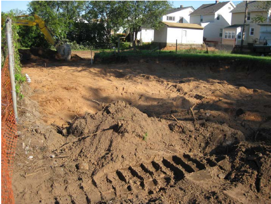
View looking East at excavated back yard
