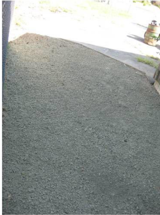
View looking East at limited excavation area being prepped for restoration
