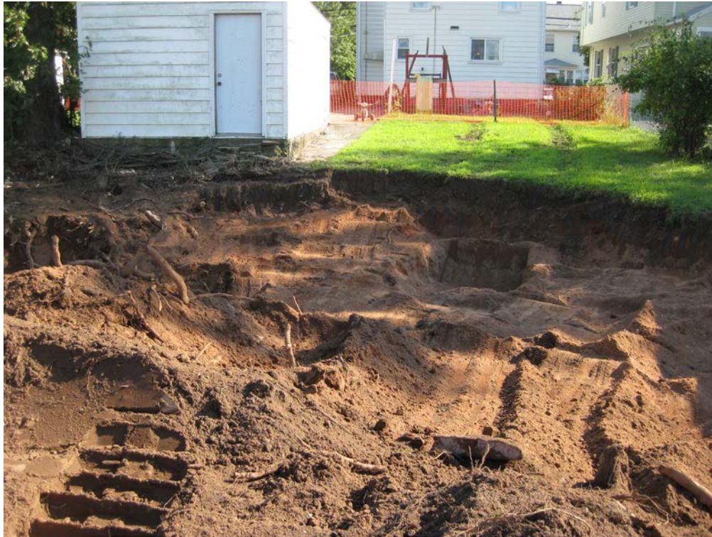
View looking East at excavated back yard
