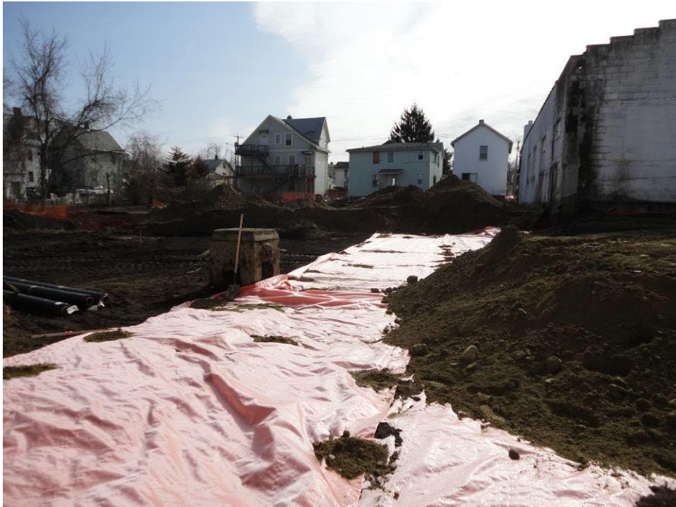
View looking East at excavated backyard following placement of marker barrier
