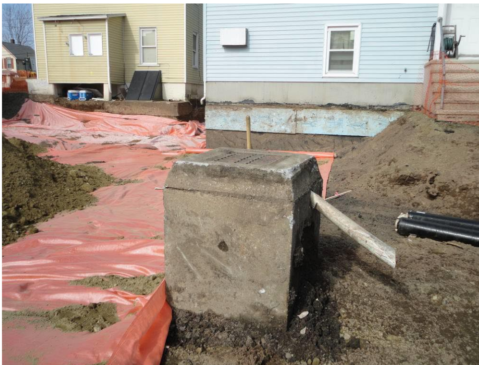
View looking northeast prior to backfilling around existing drywell
