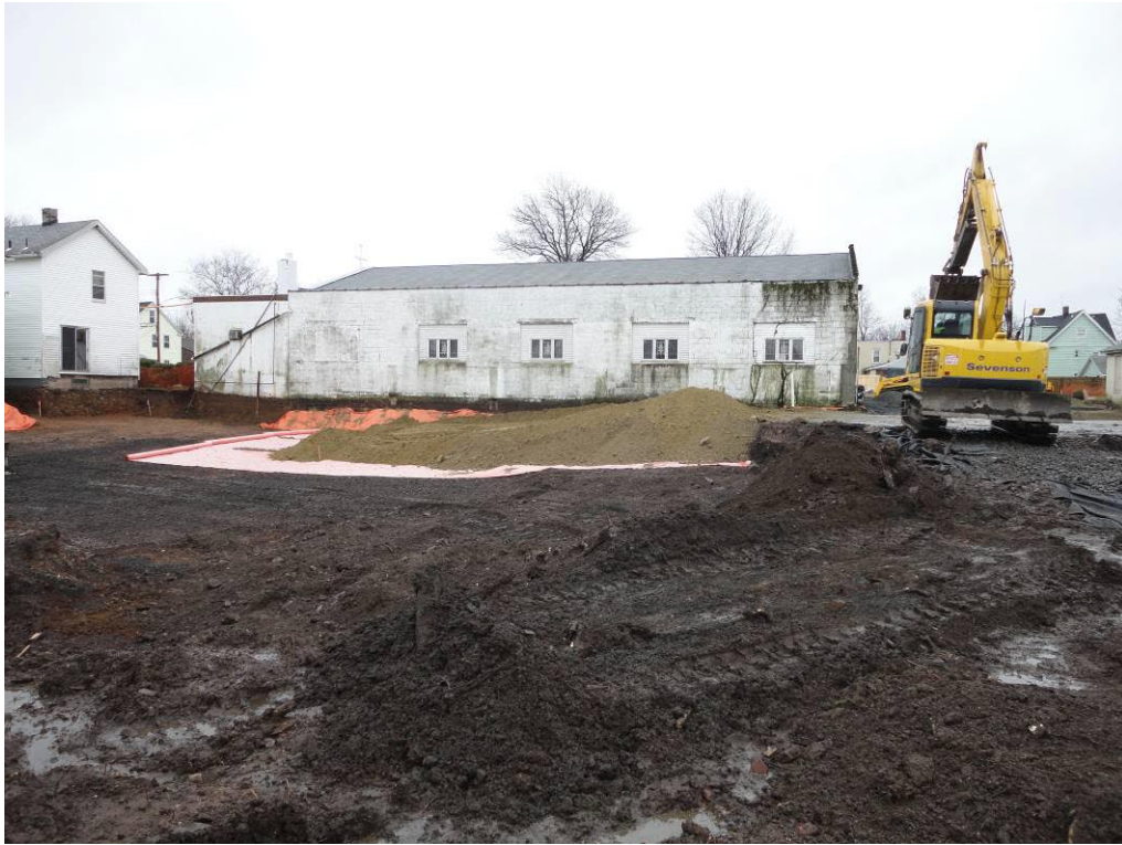
View looking South at excavated yard
