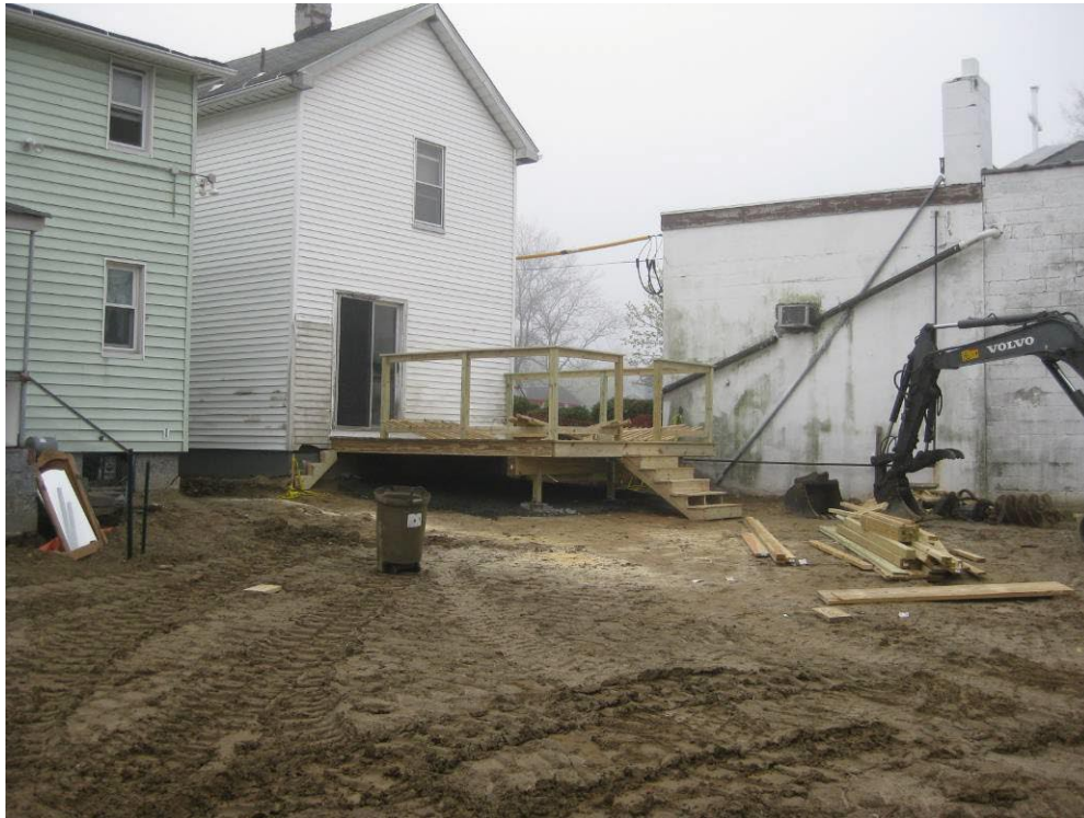
View looking Southwest at partially restored deck
