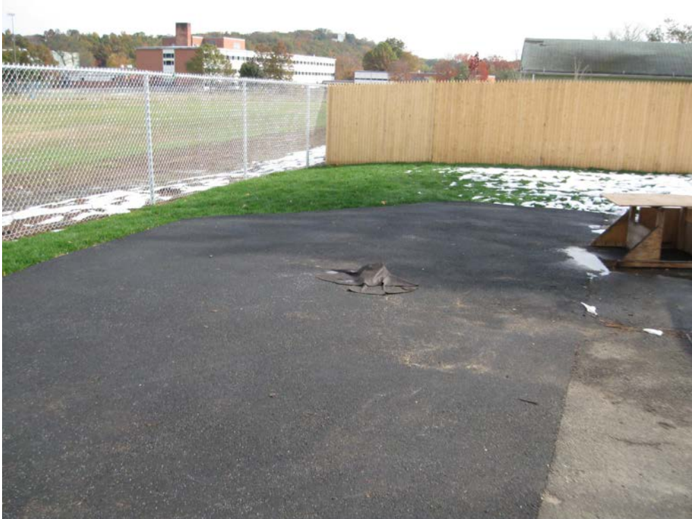
View looking East at restored back yard and parking area
