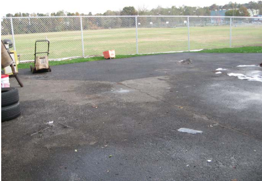
View looking North at partially restored driveway
