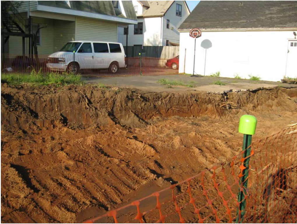
View looking Southwest at excavation of back yard
