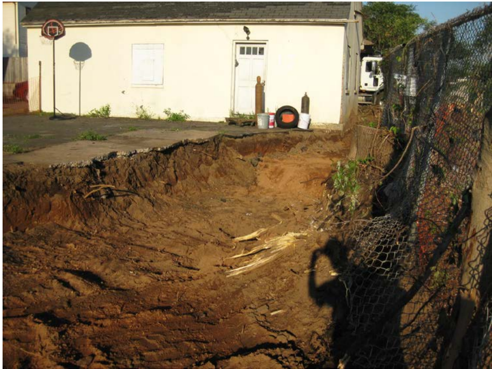
View looking West at excavation of back yard
