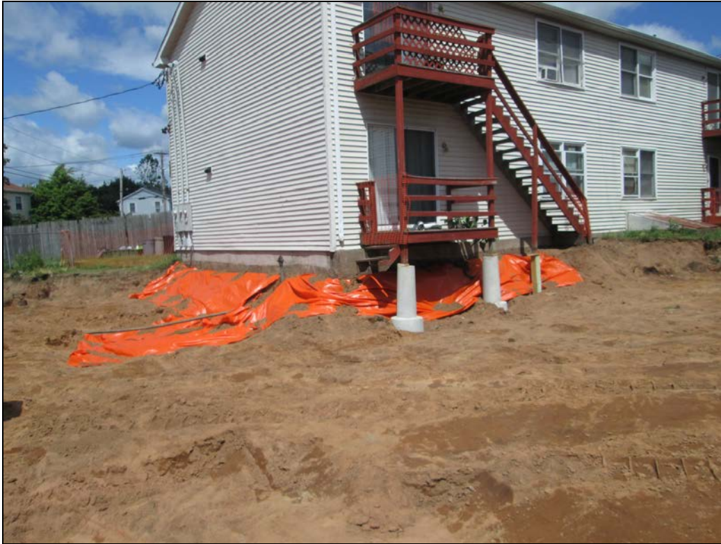
View looking northeast at excavated yard following placement of marker barrier.
