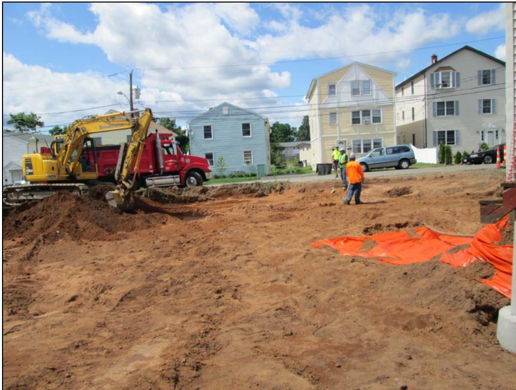
View looking north at excavated yard.
