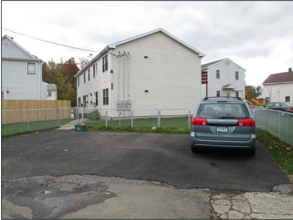
View looking south at restored driveway area.
