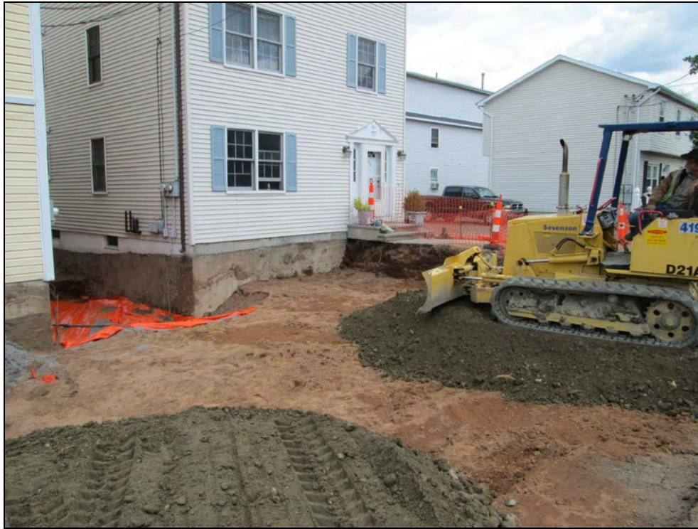
View looking northeast at partially backfilled front yard.
