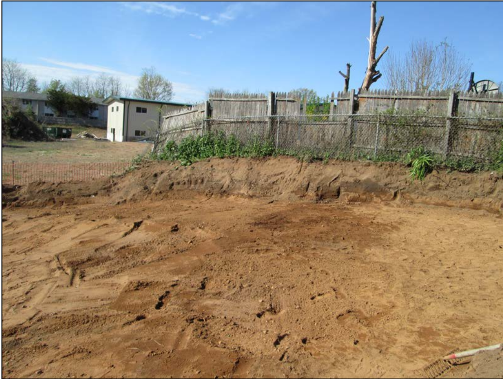
View looking northeast at excavated back yard.
