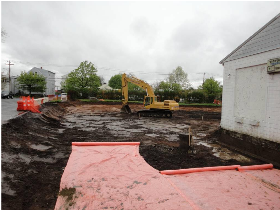
View looking North at excavated property during placement of marker barrier
