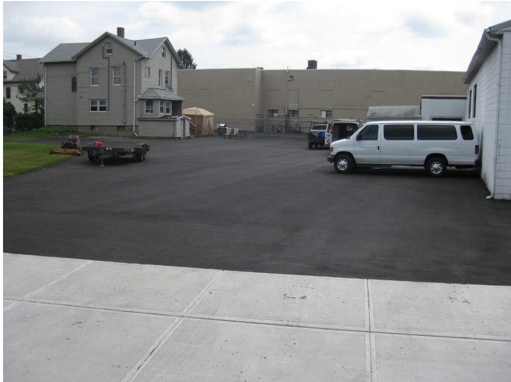
View looking East from St Mary Street at restored parking area
