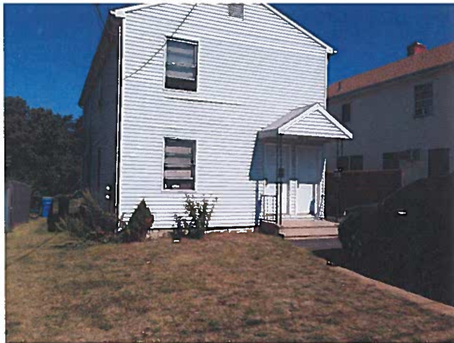
View of the Front Yard during the Fall 2014 Inspection
