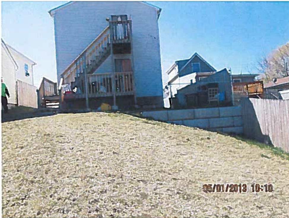
View of the Back Yard during the Spring 2013 Inspection
