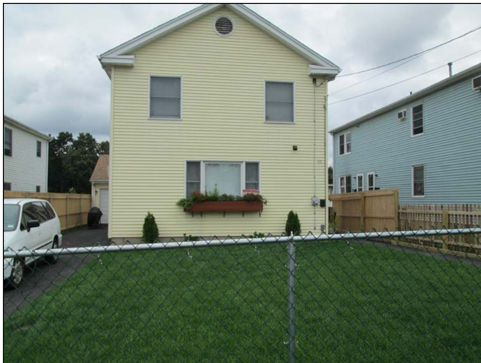
View looking north at restored front yard.
