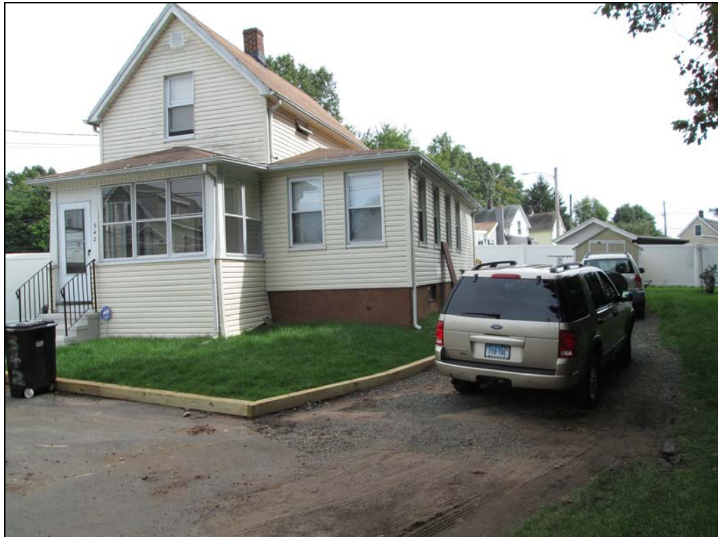
View looking south at restored front yard.
