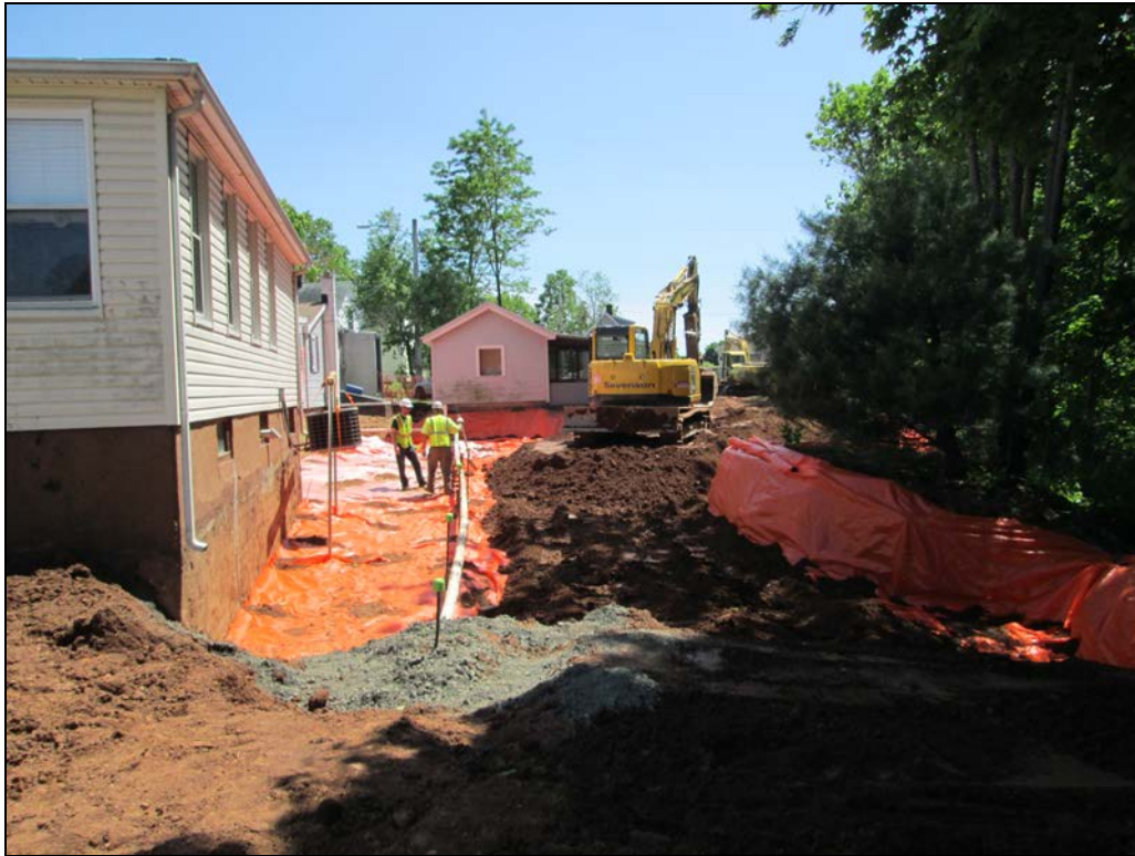
View looking south at excavated driveway area.
