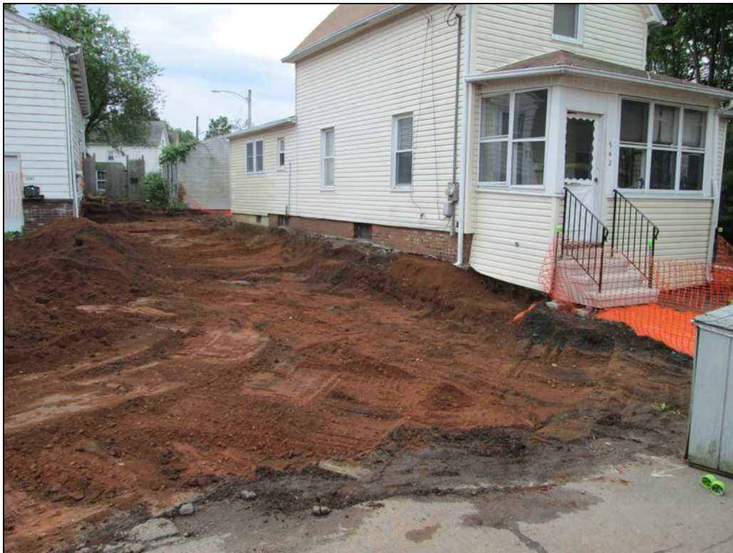
View looking southwest at excavated side yard.
