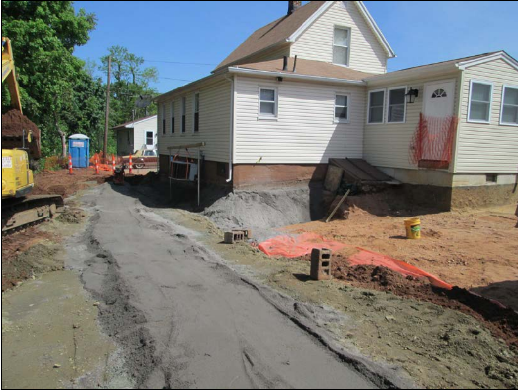
View looking north at excavated back yard.
