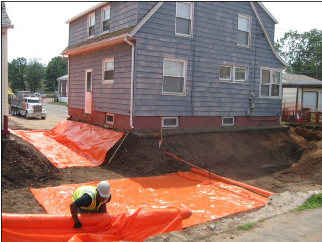
View looking southwest during installation of marker barrier.
