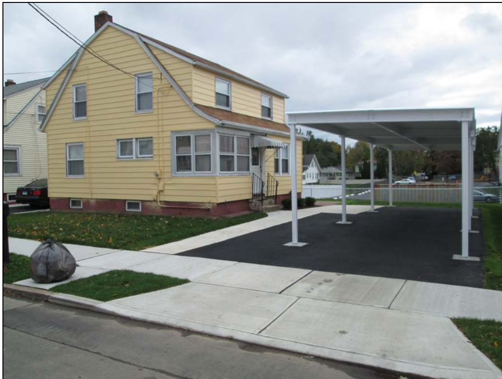
View looking south at restored front yard.
