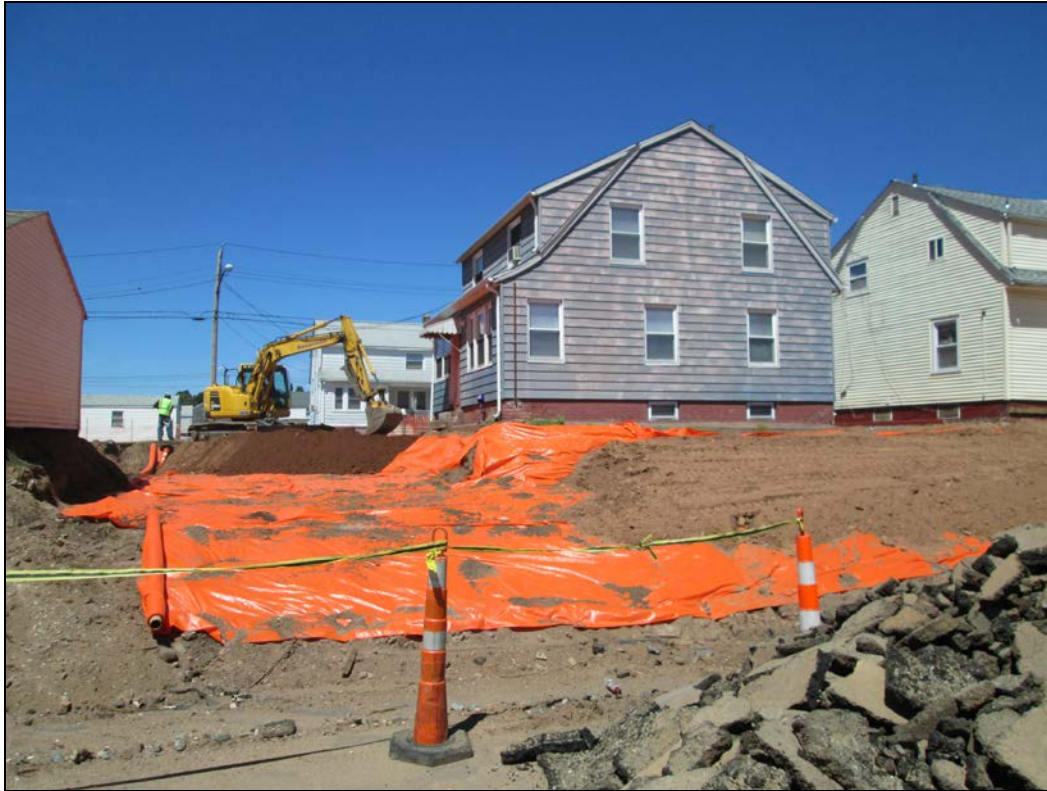
View looking north at excavated back yard.
