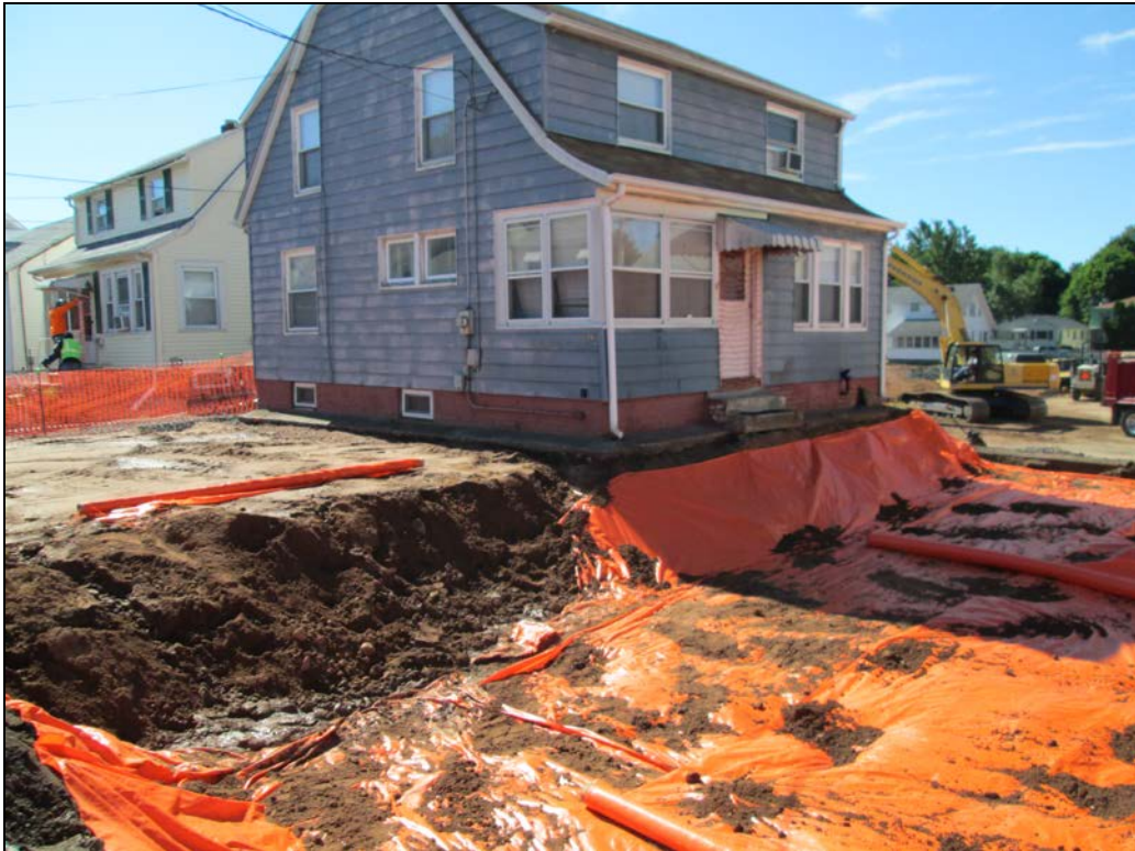
View looking southeast at excavated front yard and driveway area.
