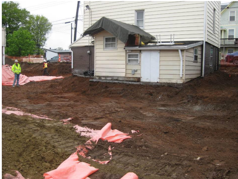
View looking West at excavated back yard
