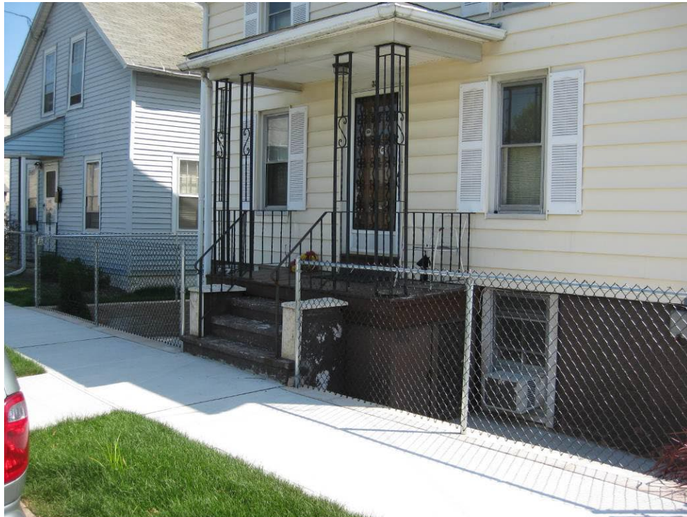
View looking Northeast at restored front of property
