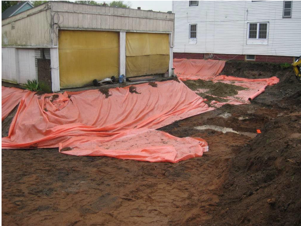
View looking Southwest at excavation around garage
