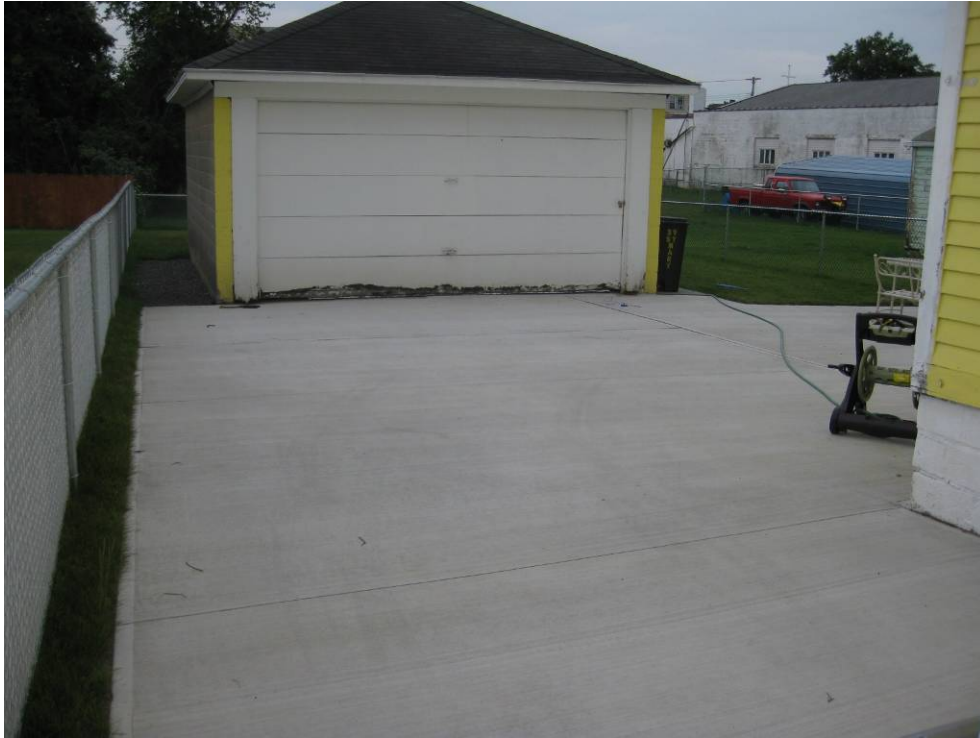
View looking East at restored driveway
