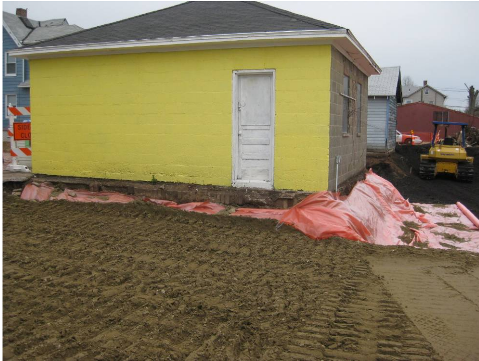
View looking South at excavation area around garage
